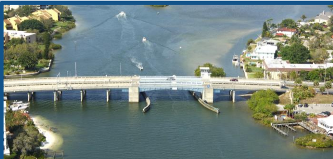
Stickney Point Bascule Bridge
