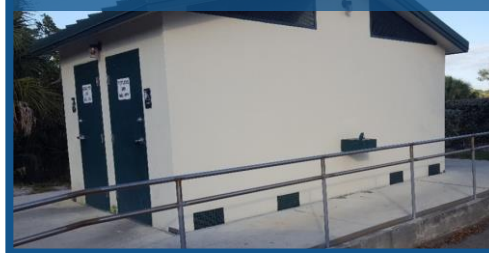
Flood Vents on a Park Restroom
