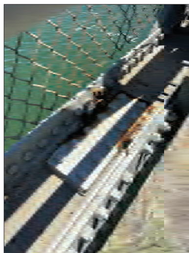
Prior truss repairs exhibiting corrosive section loss
