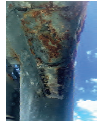
Photographs representative of existing conditions of the swing bridge's main lower truss members
