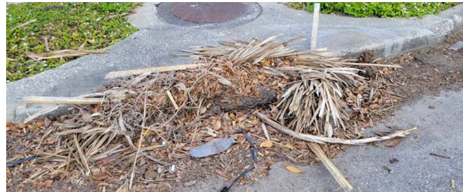
▲ Remove sediment and debris from stormdrains before they can clog pipes, cause flooding, or create sediment and litter problems in your pond | David Shafer.
