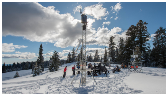
Ground-based generator PHOTO COURTESY IDAHO POWER COMPANY
