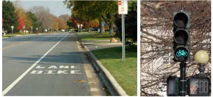
Potential bike lanes on Fox River Drive and signalized bike crossings at Route 34.
