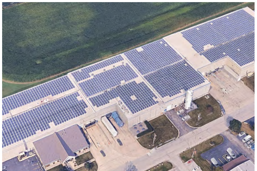
Roof-mounted solar panels in Beecher, IL
