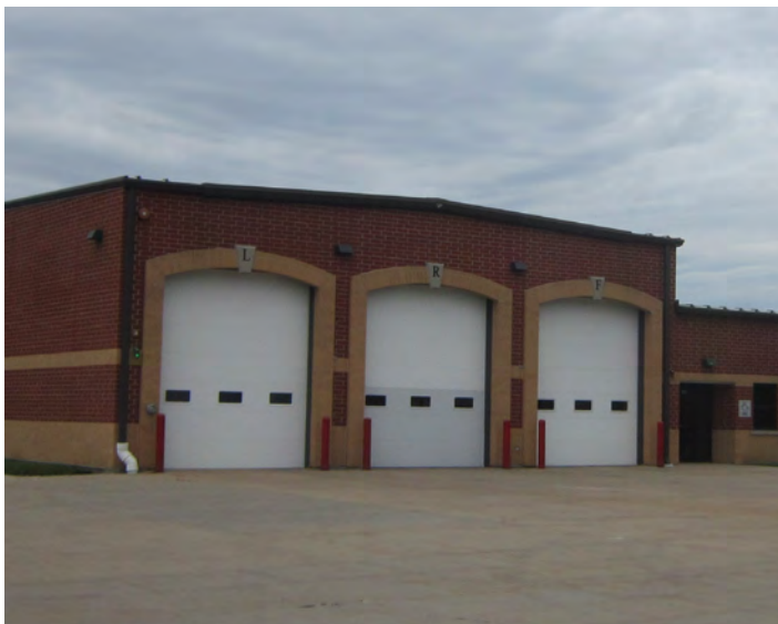
Little Rock-Fox Fire Protection District Station #3
