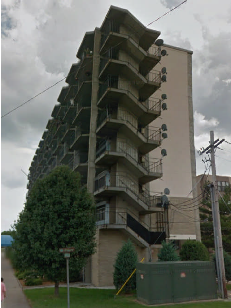
Figure 2 – 4: Smith Building East Elevation
