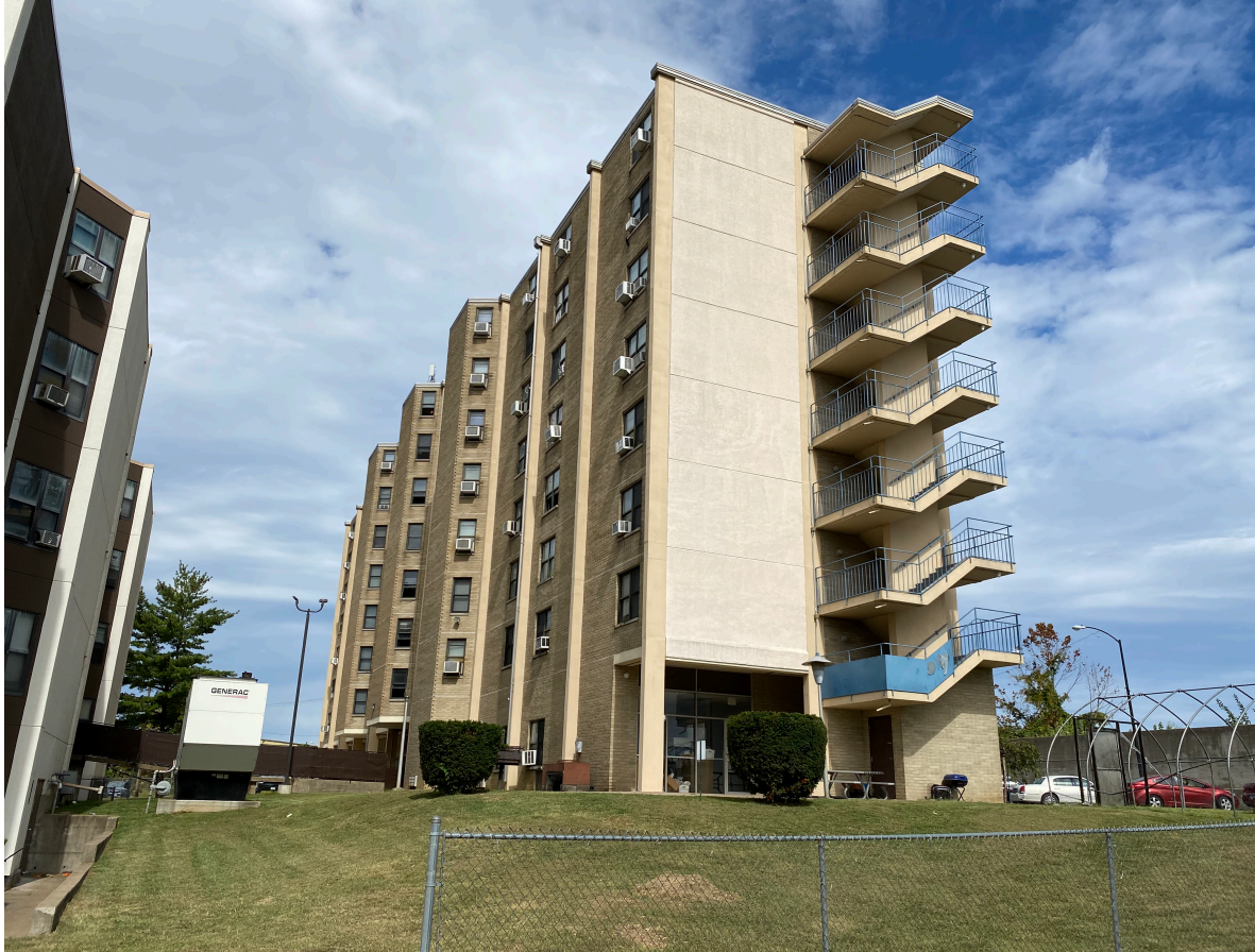
CONNEL F. SMITH BUILDING/IL-7-4 1101 Ohio St. Cairo, Illinois
