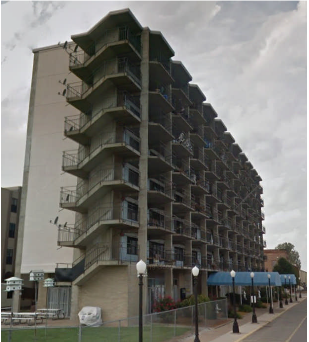
Figure 2 – 2: Smith Building East Elevation
