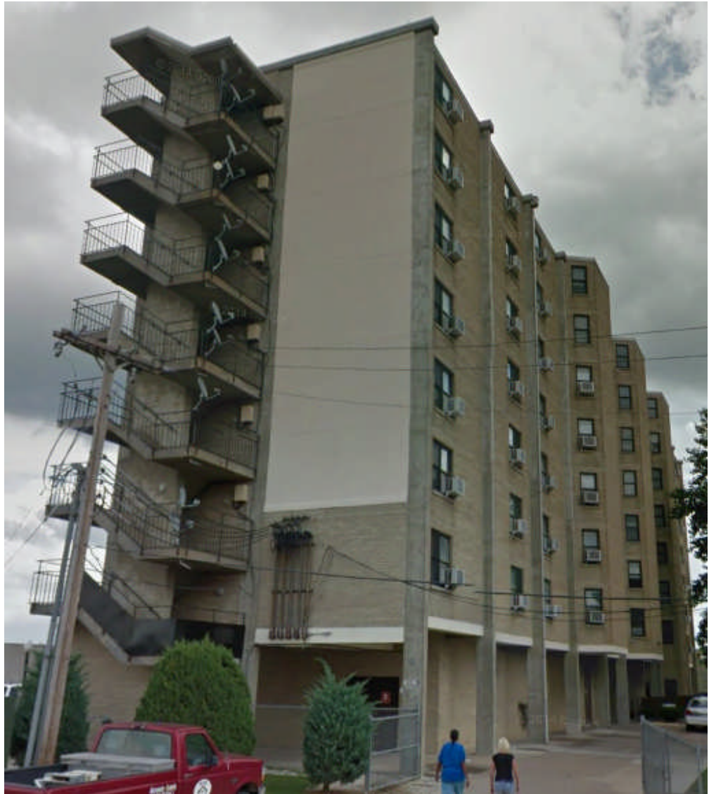
Figure 2 – 3: Smith Building South Elevation
