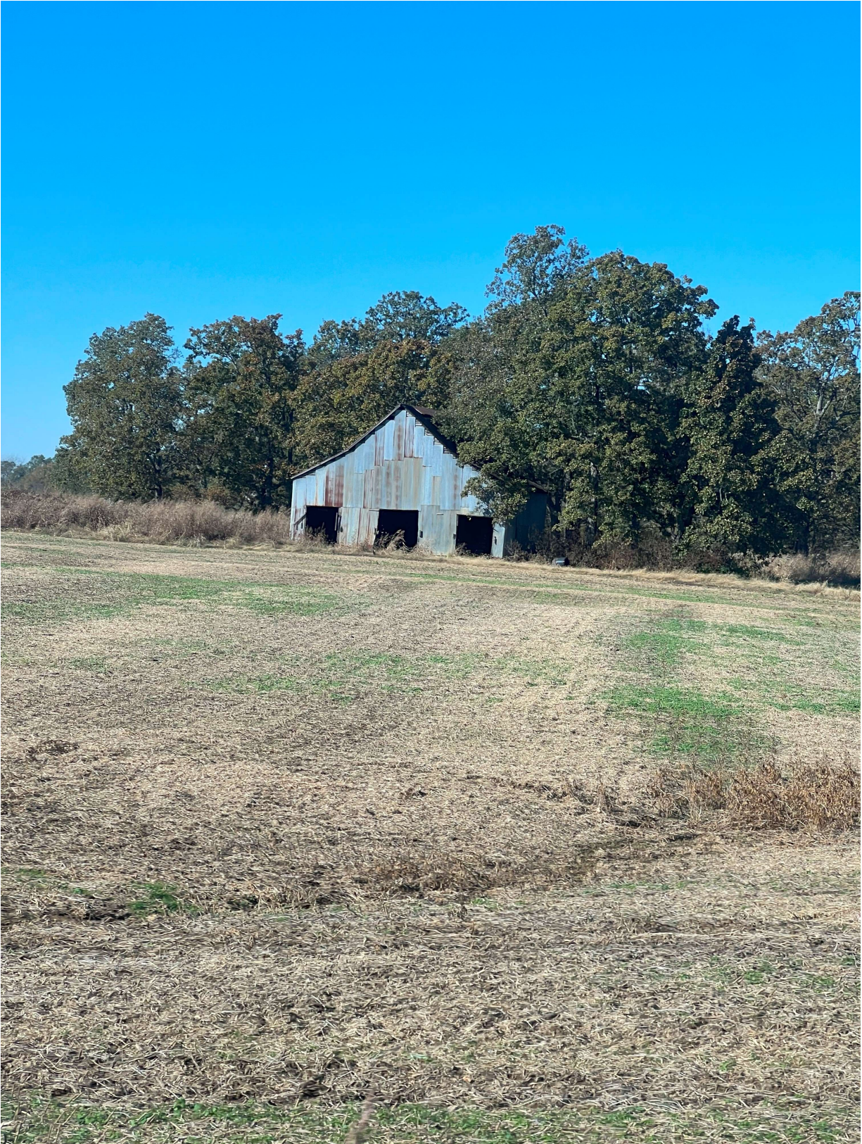
Picture (17) Stop #2 (Existing barn #2 to be removed)
