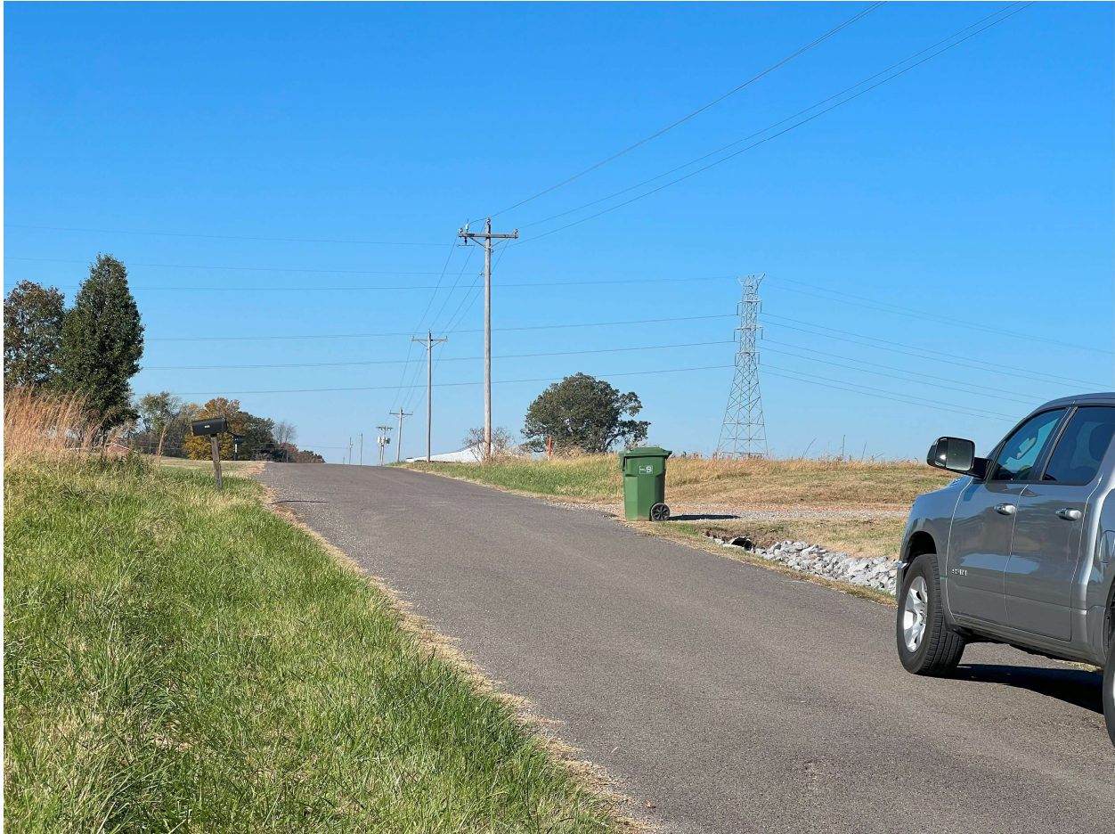
Picture (10) Stop #1 (Looking at Transmission Line)
