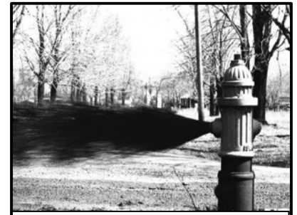
City of Oneida hydrant being flushed. Circa 1930s.
