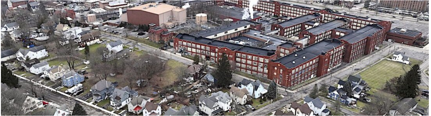
The former Remington Arms complex today: vacant, deteriorating, and in the center of the Village.
