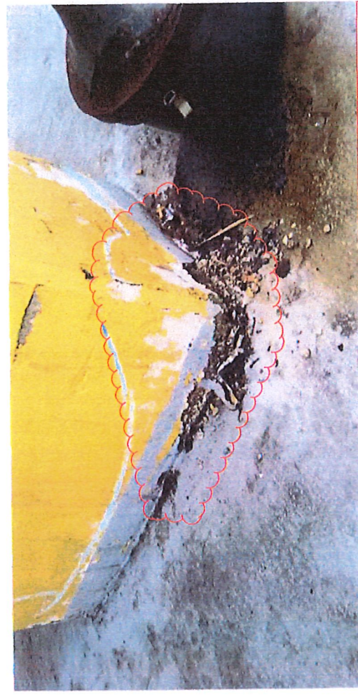
1.3 Deteriorated Column Base
