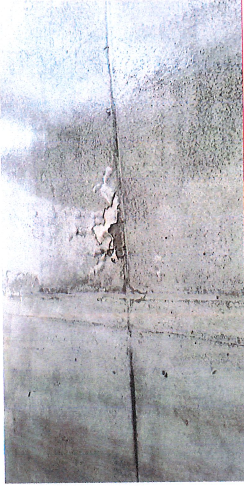
3.2 Failed Membrane
