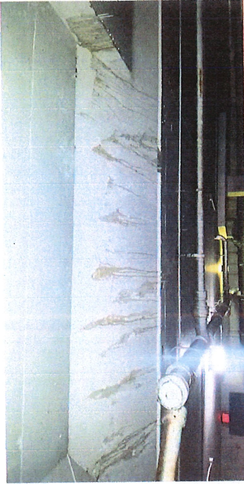
4.2 Underside Plaza Leaking
