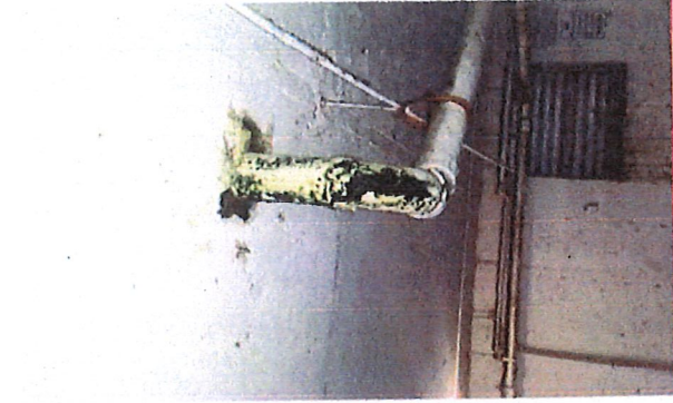
3.3 Leaking Drain
