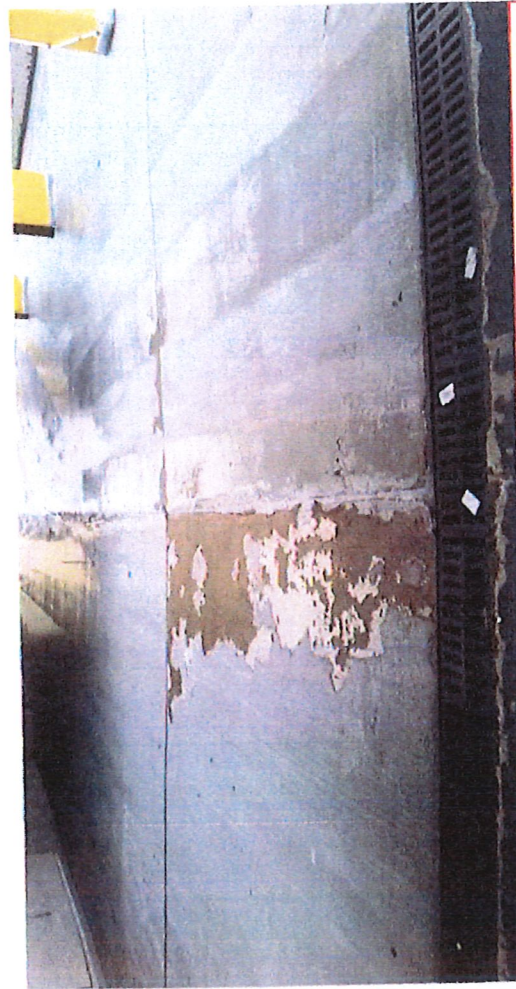
2.3 Failed Membrane
