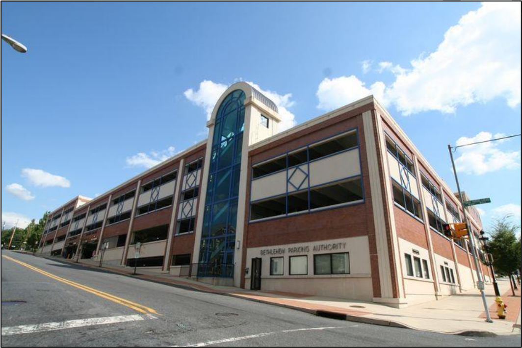
North Street Garage
