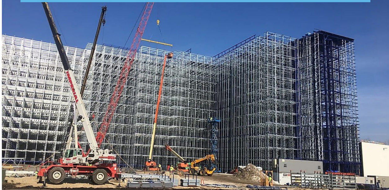
The 130-foot-tall Americold Rochelle Automated Storage and Retrieval System under construction in Rochelle, Illinois (above) and completed (below). Photos courtesy of Griffco Design/Build, Inc.
