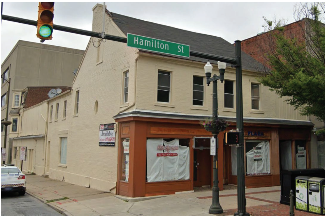
Fig. 6: Front and side elevations of the building at 10 th and Hamilton Streets, 2019. (Google StreetView)
