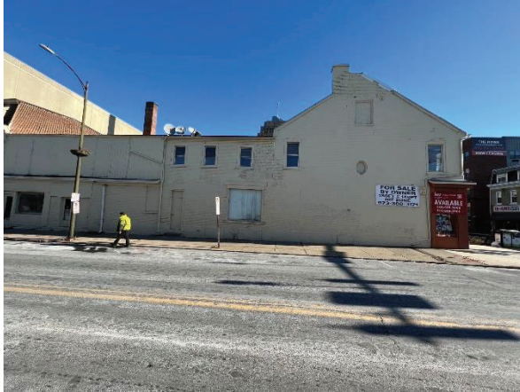
Photo #7 – 10 th Street Façades
