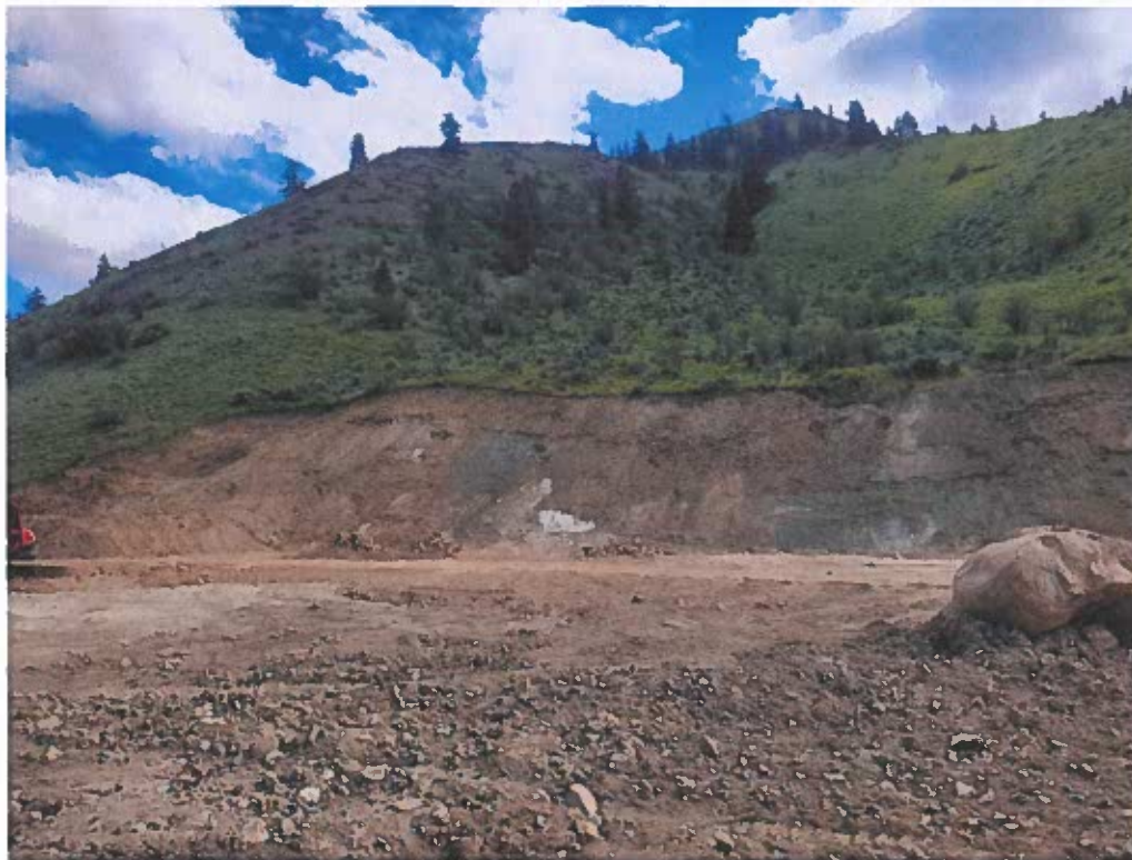
Figure 1.4 Cut slope south of proposed building location
