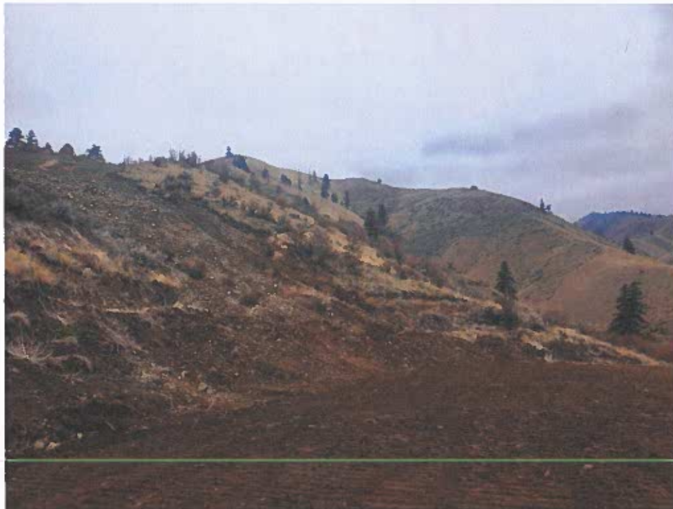
Figure 4 Cut slope south of building pad on Parcel 222007000100
