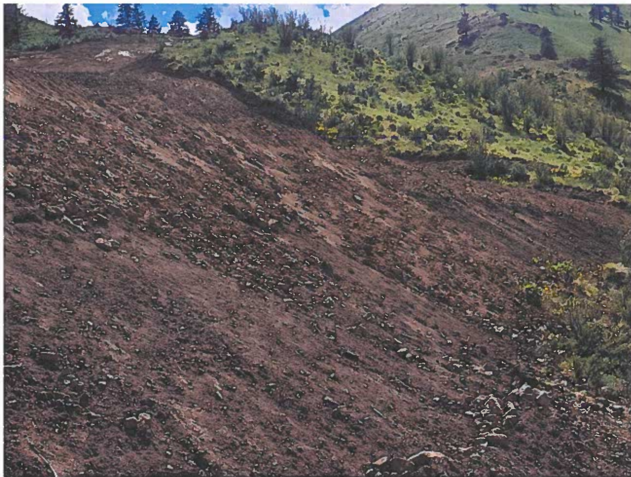
Figure 1.5 Fill slope north of proposed building location
