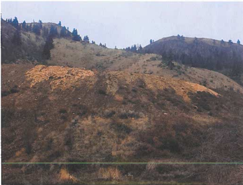
Figure 6 Straw ground cover on southerly fill slope
