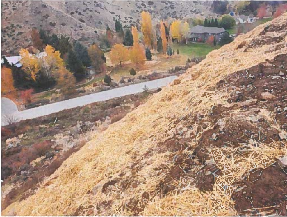
Figure 5 Straw ground cover on southerly fill slope
