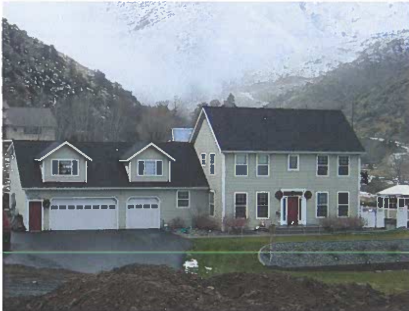
Figure 1.3 Single-family home on adjacent property to the north
