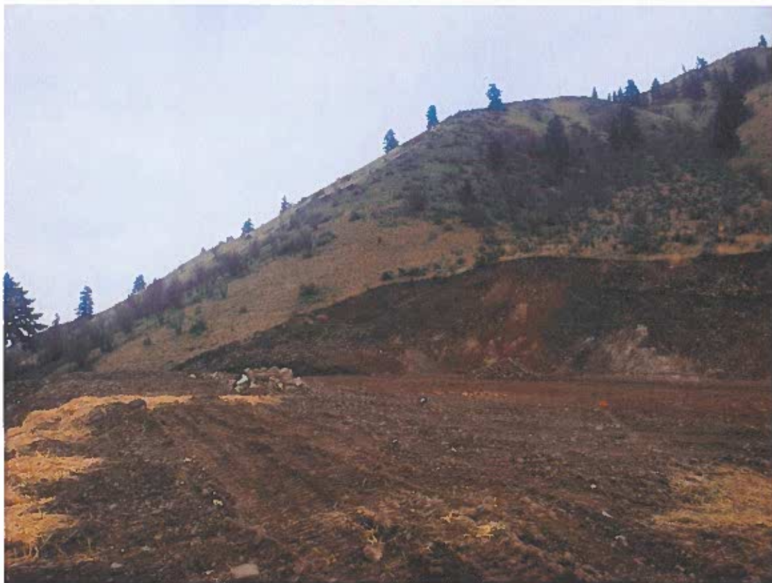
Figure 2 — Cut slope south of building pad on Parcel 222007120050
