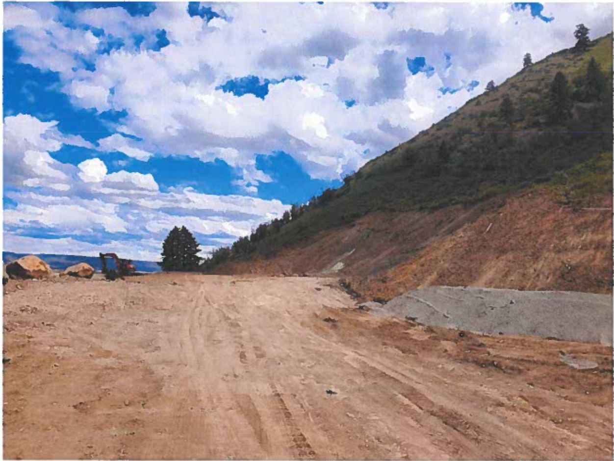
Figure 1.2 Slope east of proposed building area
