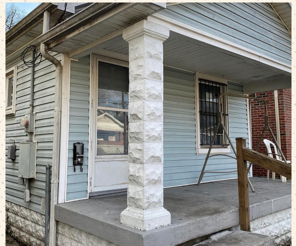
Cast concrete porch columns and foundations are typical throughout Louisville's West End, including the Algonquin and Park Hill neighborhoods.
