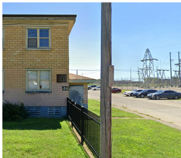
Several apartment buildings are directly adjacent to the LG&E transmission station.
