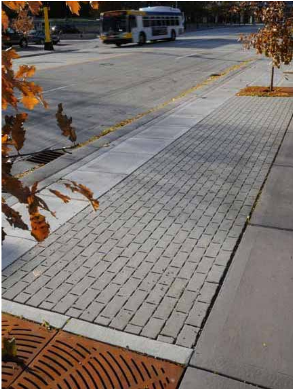
PERVIOUS PAVERS BETWEEN TREE WELLS WILL INSURE INFILTRATION OF WATER FOR THE TREES
