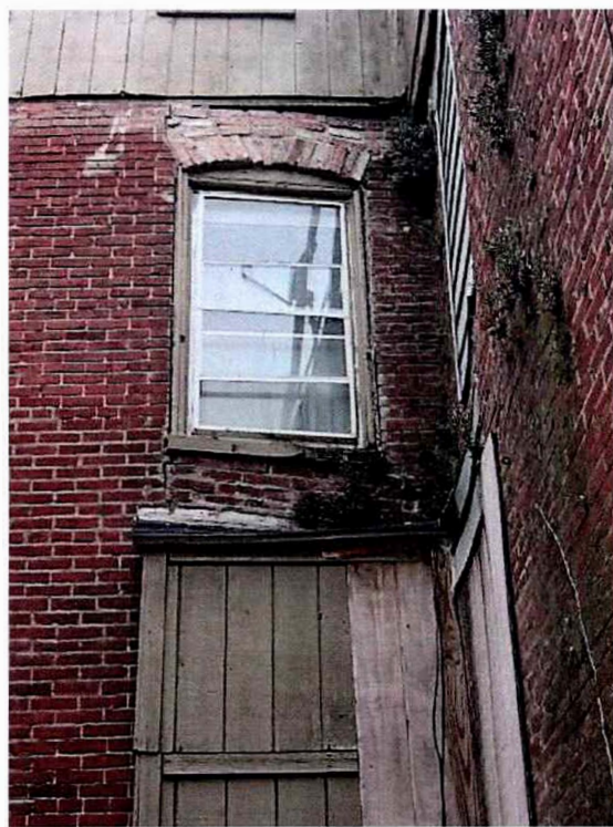
Photo 4 – Wall displacement along east face window
