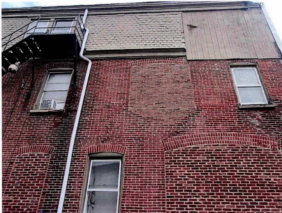
Photo 8 – Wall displacement/cracks
