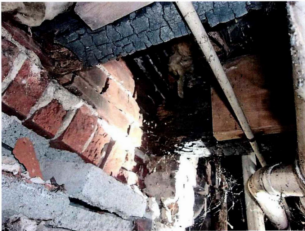
Photo 16 – Unsuitable bearing of framing at fire damage
