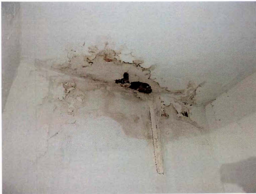
Photo 19 – Signs of rainwater infiltration at interior space
