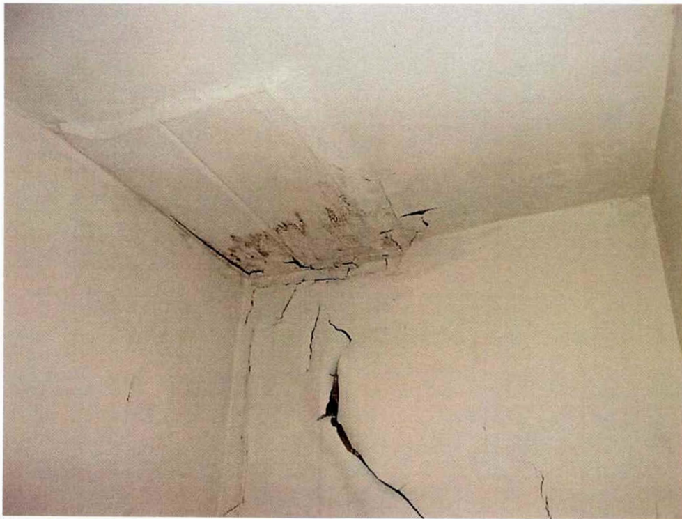
Photo 21 – Signs of rainwater infiltration at interior space
