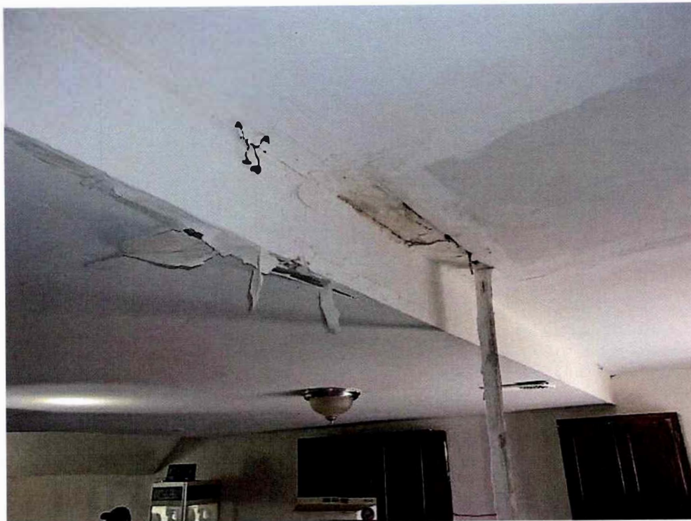
Photo 20 – Signs of rainwater infiltration at interior space
