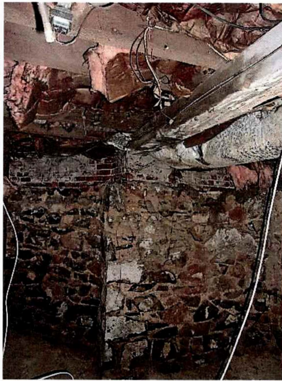
Photo 14 - Floor framing member lacks end support
