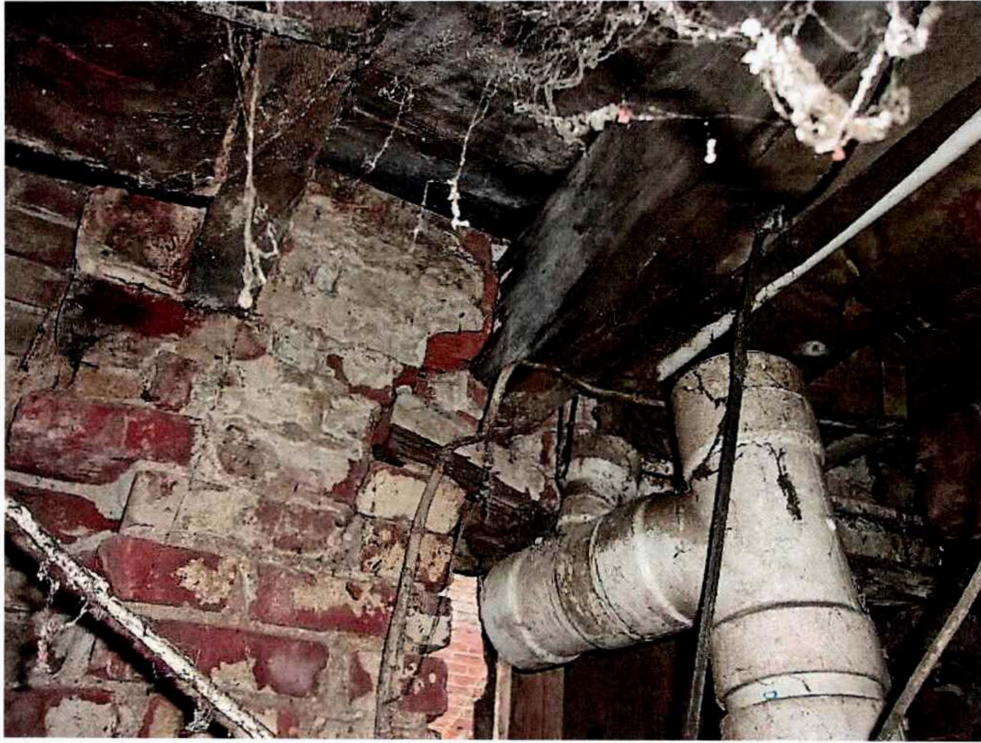
Photo 13 – Unsuitable wall bearing below floor joist
