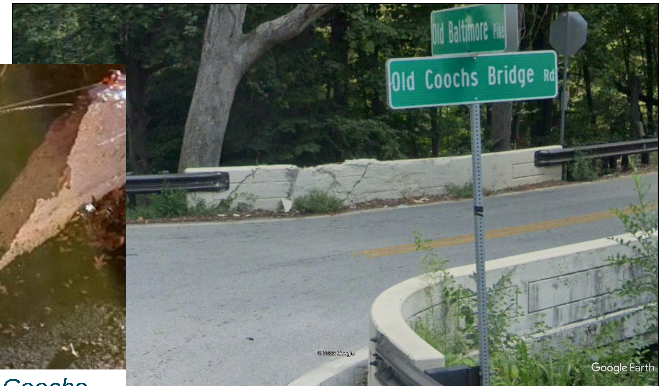
Bridge 1-337 Old Coochs Bridge Road: NB Parapet Vehicle Impact January 2023
