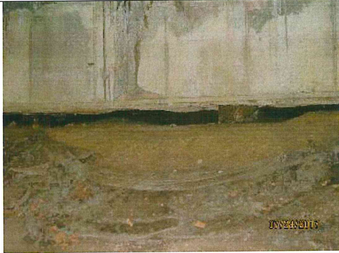
Photo 4: Exposed piles.
