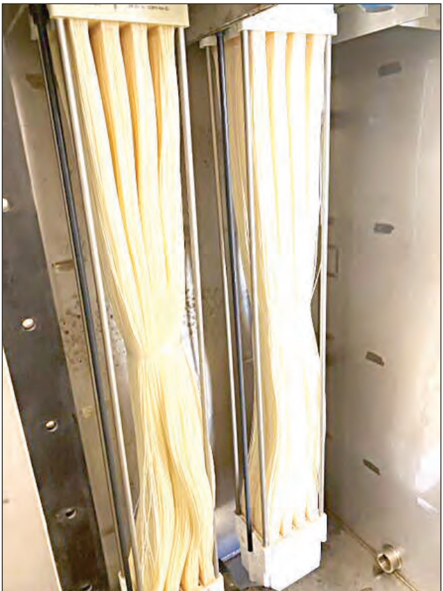
PHOTO PROVIDED BY UNDERWOOD ENGINEERS Veolia hollow fiber membranes are part of the wastewater treatment project servicing the facilities at the Mount Washington summit.
