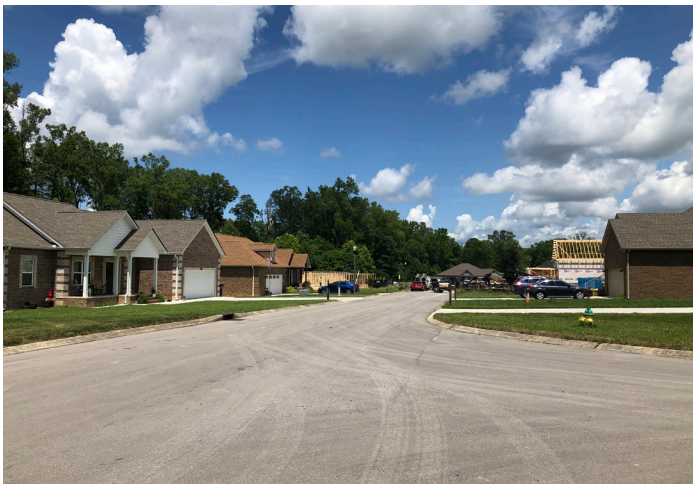
This new Tullahoma subdivision lacks some of the design features that are recommended for future design standards at right, including sidewalks and street trees.
