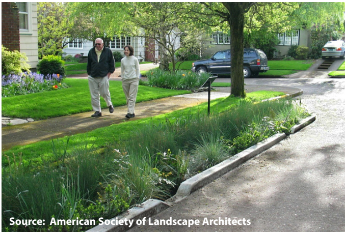
Bioswales can be installed between a street's curbing and the planting strip. They are designed for stormwater to drain into them so the water can be absorbed into the soil and plant materials to protect the more conventional drainage systems from being overwhelmed.
