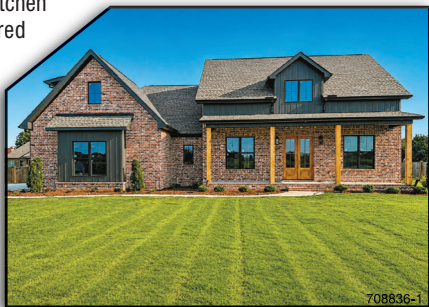
NEW CONSTRUCTION CORNELIUS LANDING
