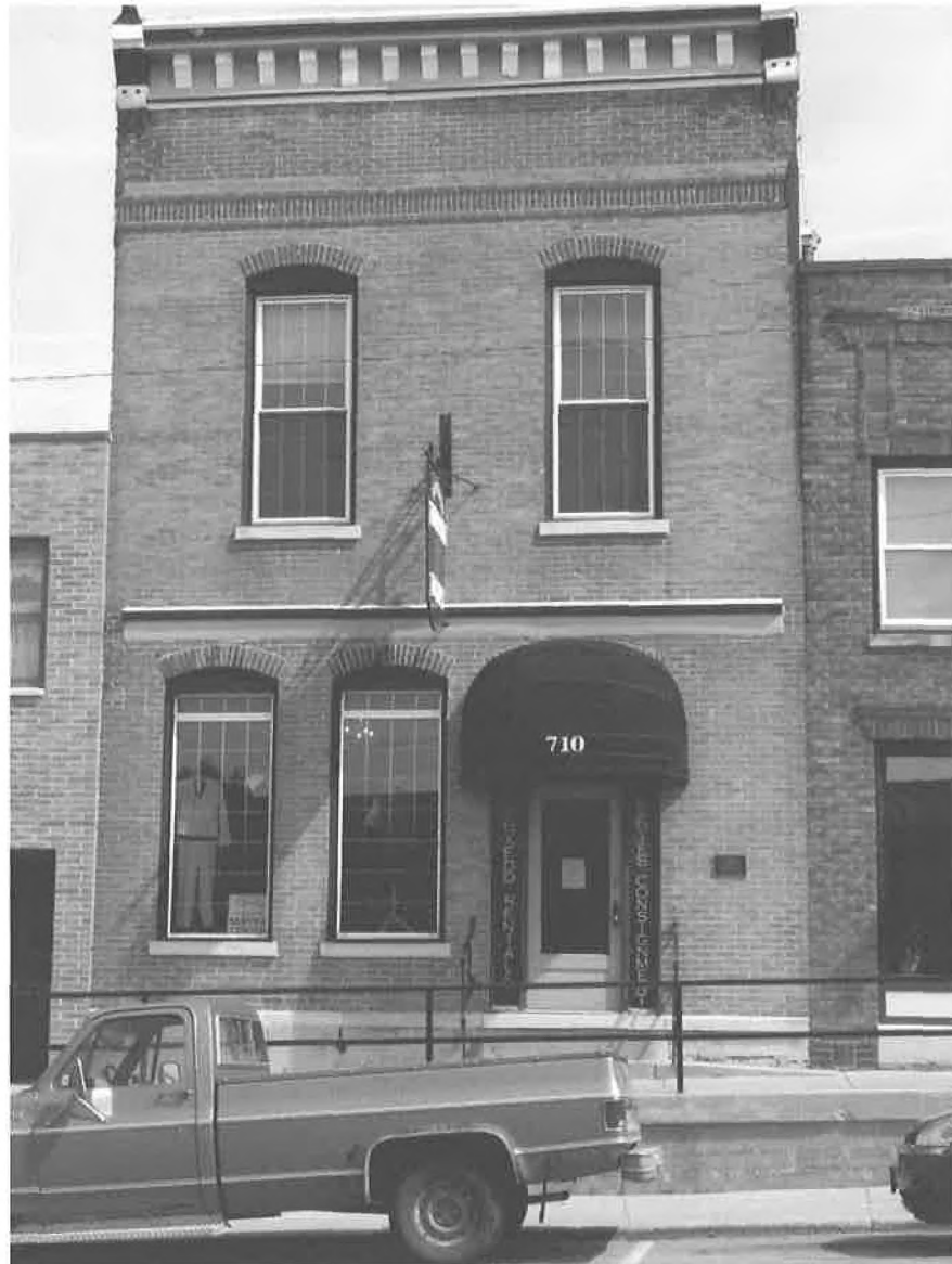
Figure 16 Women's Relief Corps (WRC) Hall (NRHP), 710 Washington, 2009 photo
