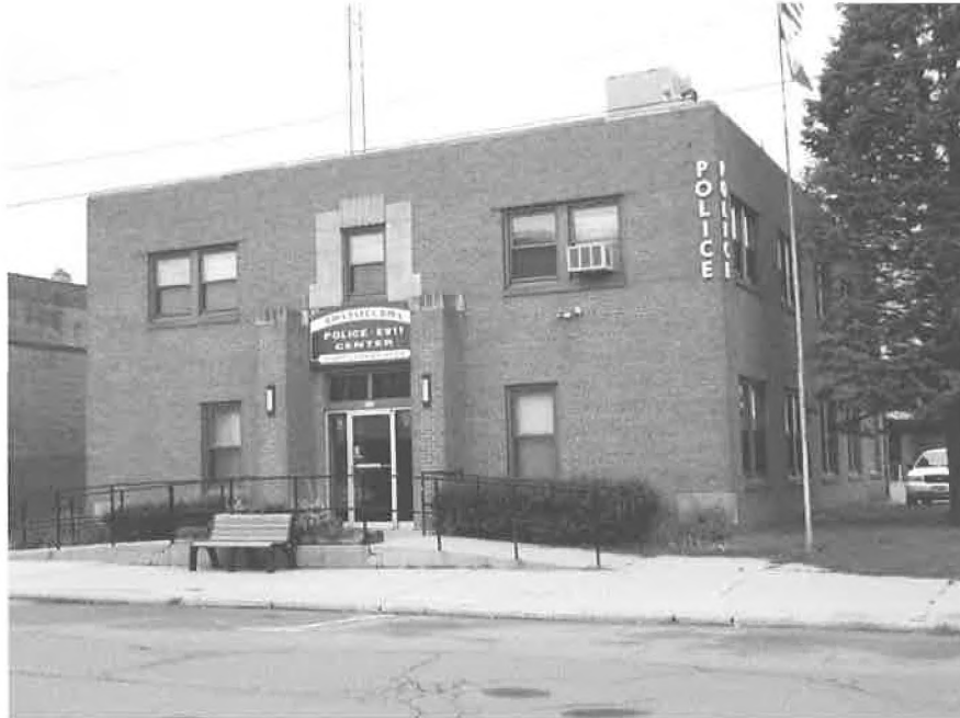
Figure 30 City Hall, 321 Stevens, 2011 photo
