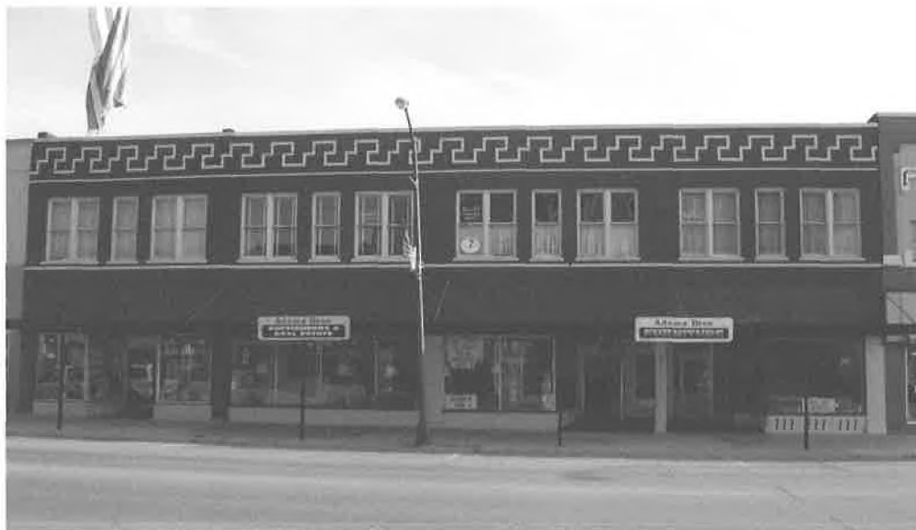
Figure 25 Cuplin Block, 2009 photo Note addition of matching storefront on left
