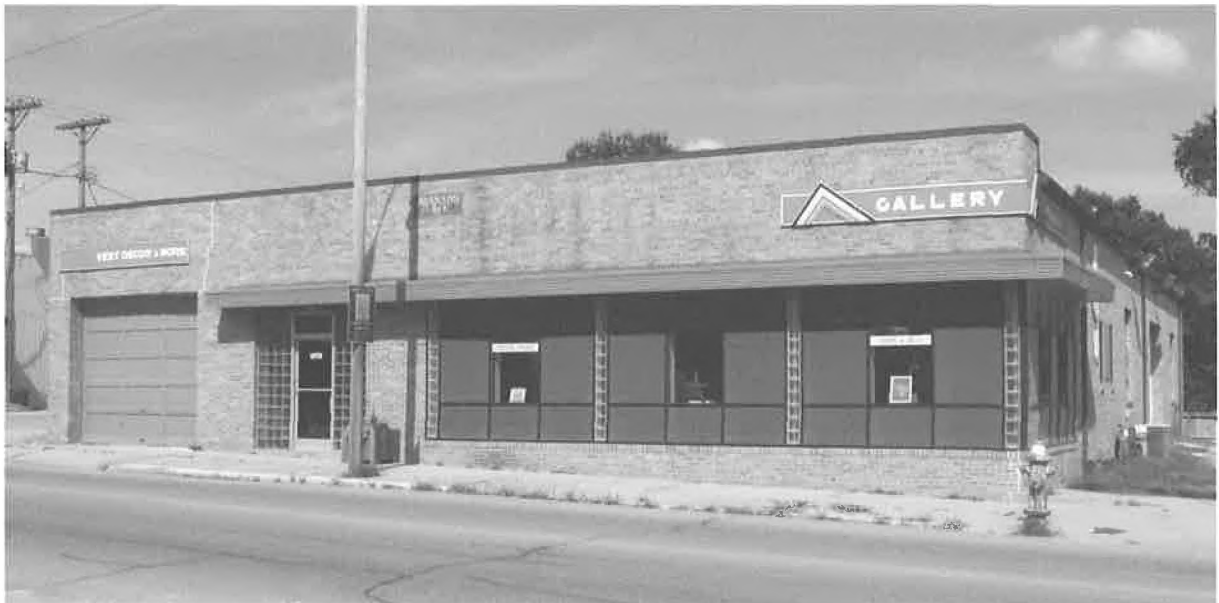
Figure 35 Central Motors, 202 Oak, 2009 photo
