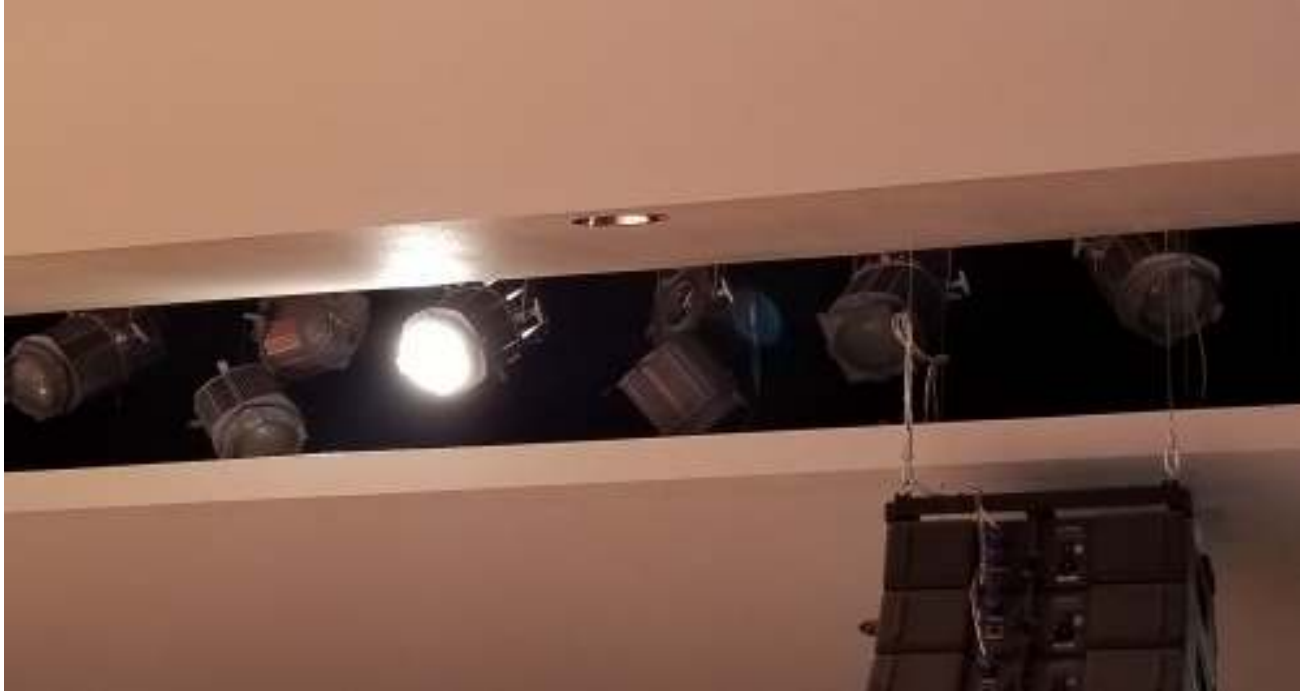
Image shows front light mounting location and only one of every six fixtures working.
