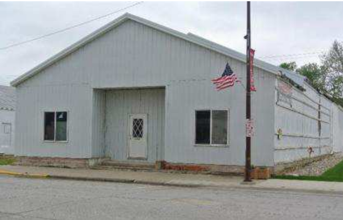
1109 Water Street, Alden, Iowa
