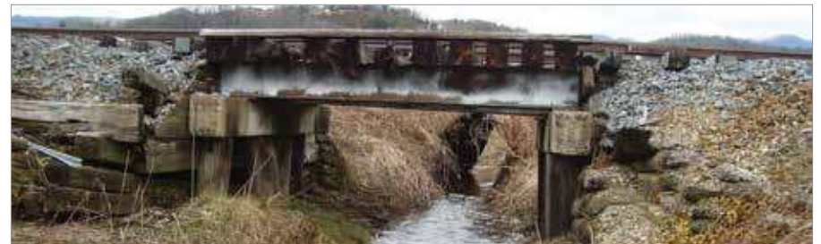
Typical Minor Bridge
