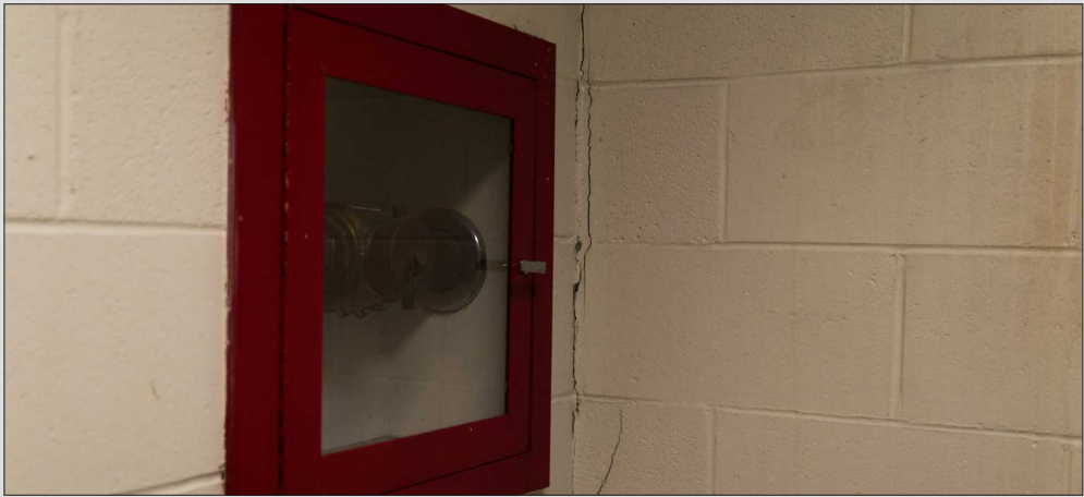
Cracks in the walls of the staircase. Sarabond, which was used in the construction of DeRoy Apartments, was found to deteriorate building structures and may cause brick to crumble, according to The New York Times. Photo by Jonathan Deschaine.
