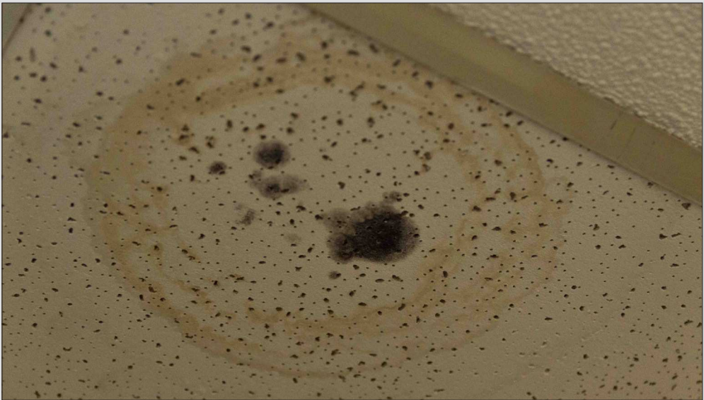
Black mold on the hallway ceiling of Deroy Apartments. Photo by Jonathan Deschaine.
