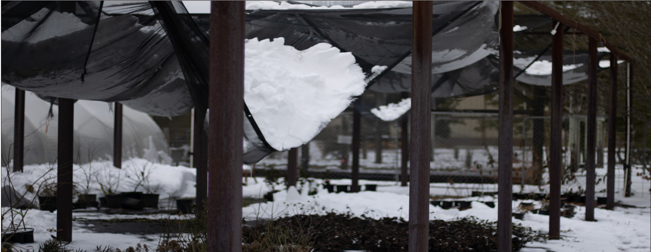
SFA Gardens suffered plant and structural damage in a snow storm in early 2021. The outdoor plants were iced over and the supporting beams were bent from the weight of the snow.
