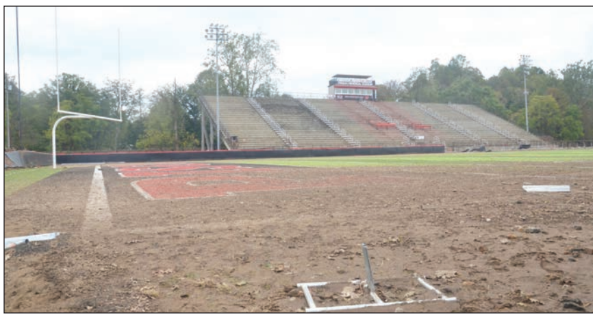
DAMAGES — Mud covered the field at Pisgah Memorial Stadium where fencing was destroyed and goalposts were twisted during flooding. Aarik Long
