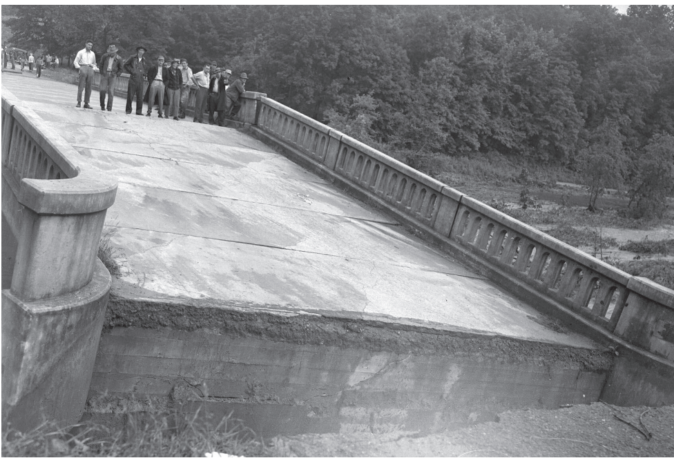
A bridge washed out by the Pigeon River flood of 1940.
