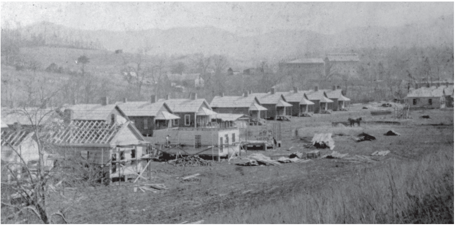
Fibreville under construction circa 1906.
