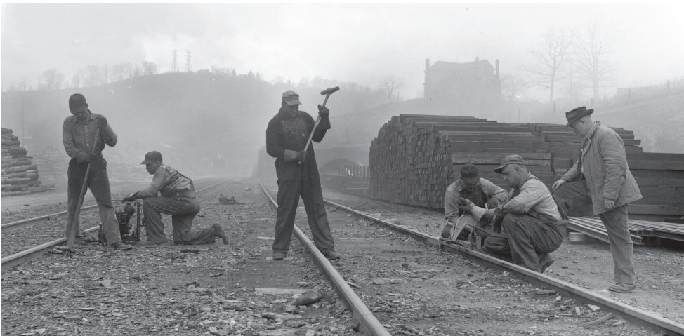
Workers along railroad tracks leading through the mill woodyard.
