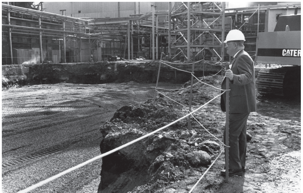
Champion officials tour progress on the $250 million modernization project in 1991.
