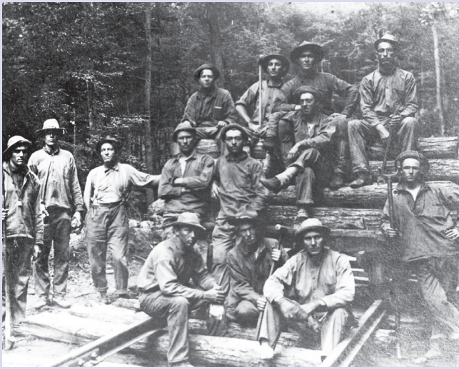
Men of the 106th Engineer Regiment came to Sunburst during WWI to train on building bridges and trestles in the war effort.
