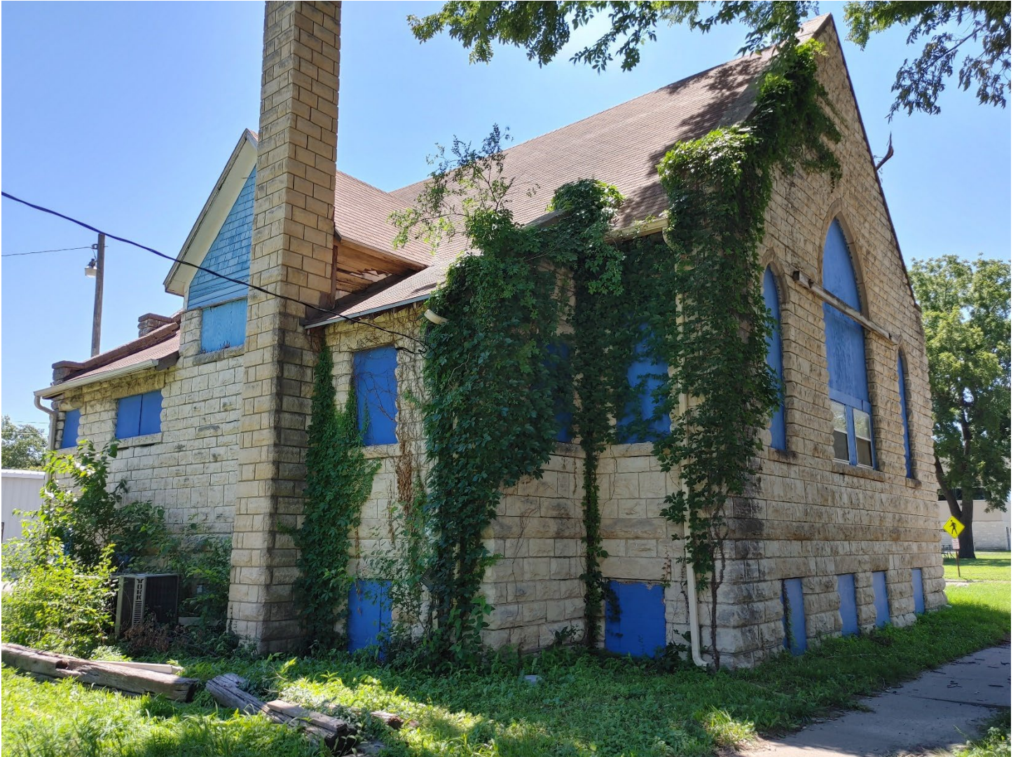
Photo 2: Shepard Chapel, NW corner, camera facing SE
