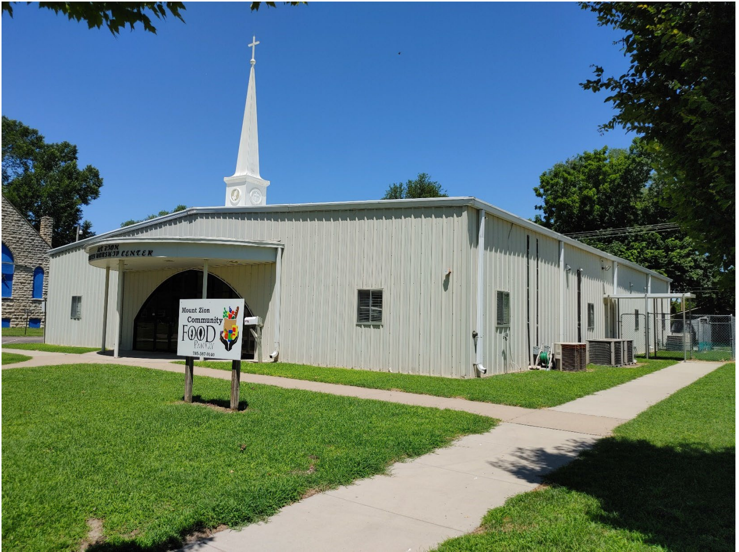
Photo 7: Mt Zion, SE corner, camera facing NW
