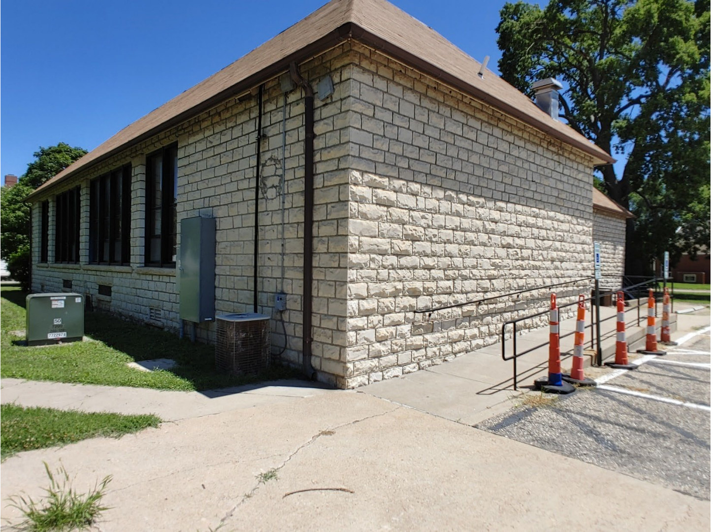
Photo 13: Douglass School, SW corner, camera facing NE
