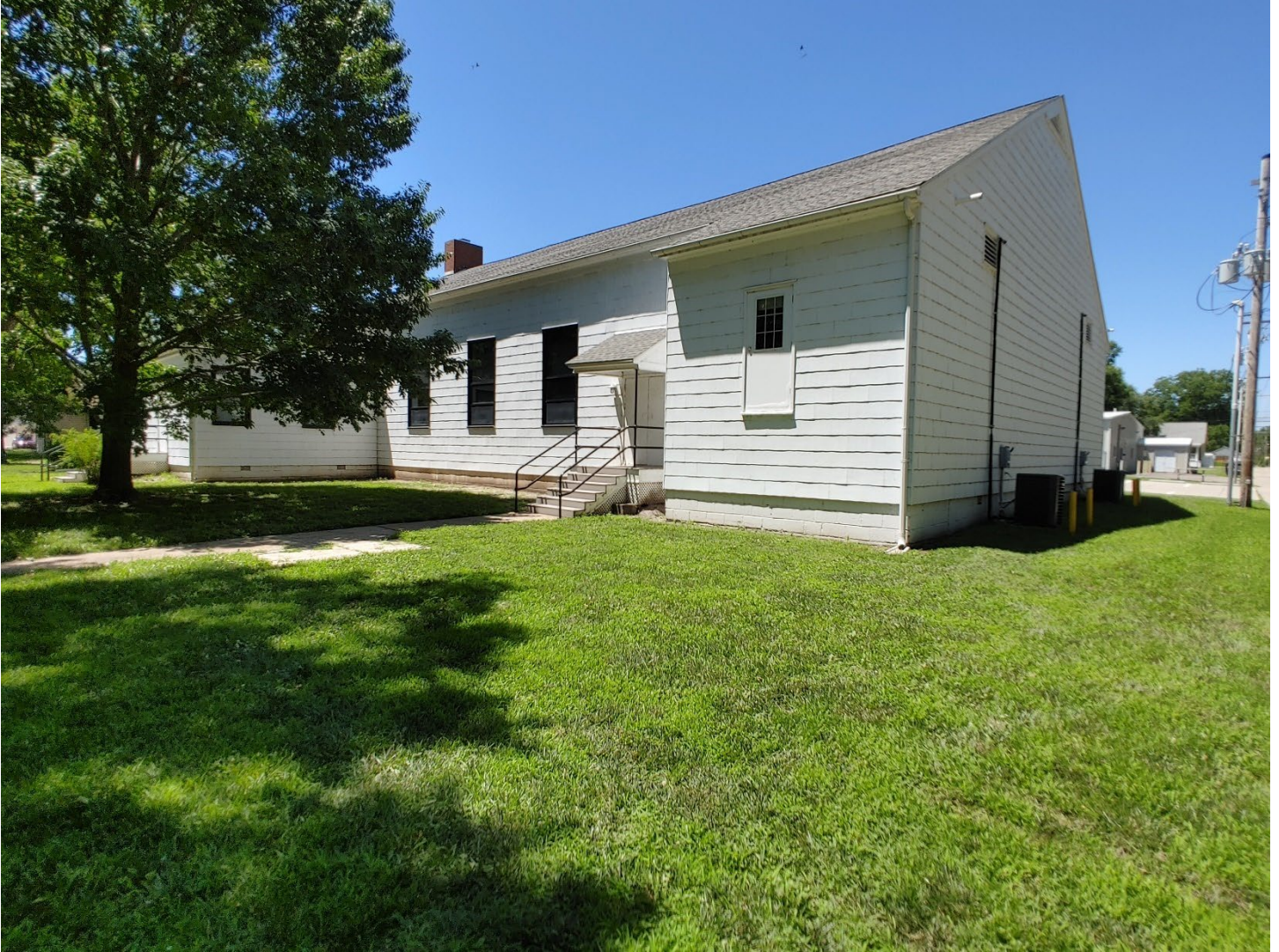
Photo 16: Douglass Community Center, NE corner, camera facing SW
