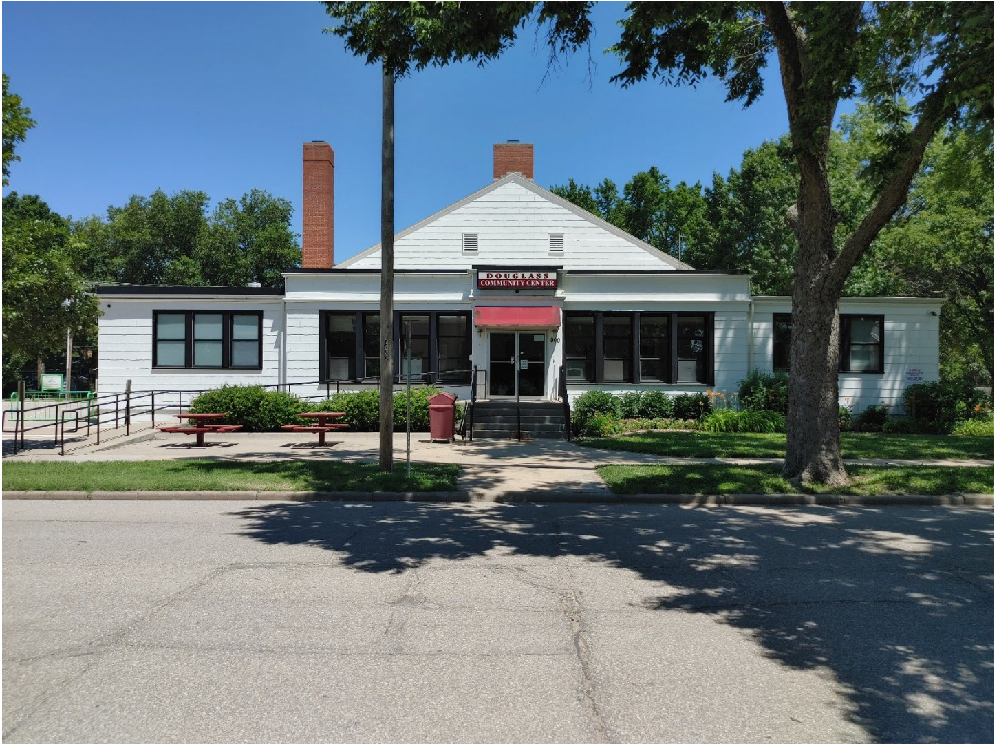
Photo 18: Douglass Community Center, S façade (front of building), camera facing N
