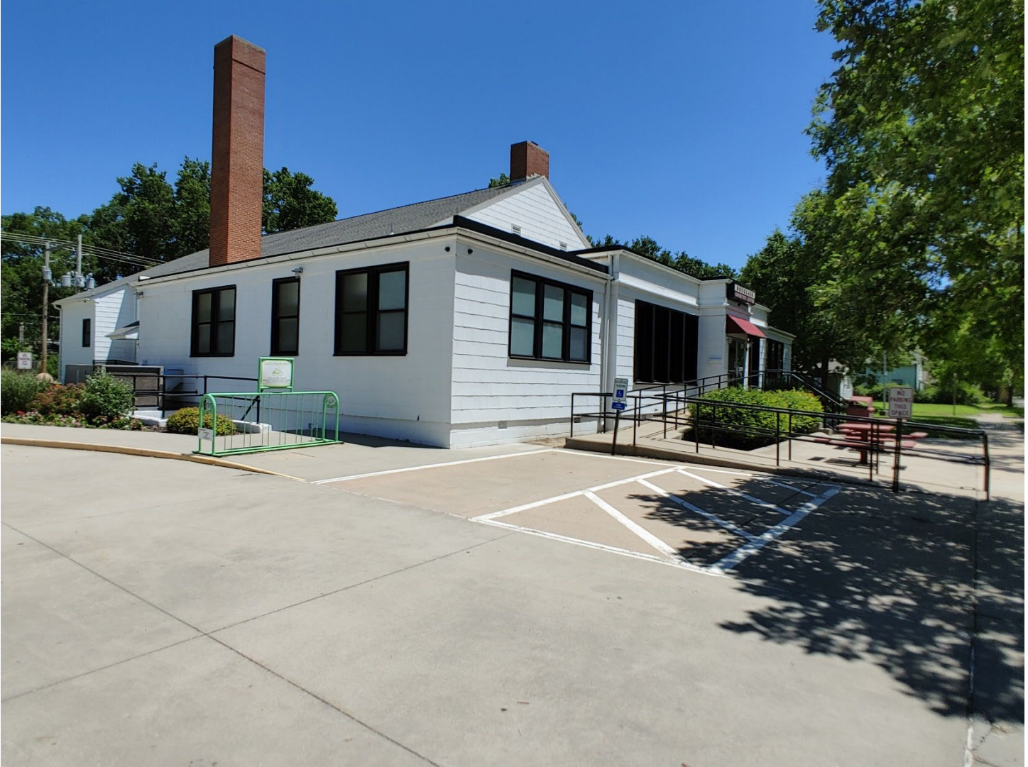
Photo 14: Douglass Community Center, SW corner, camera facing NE
