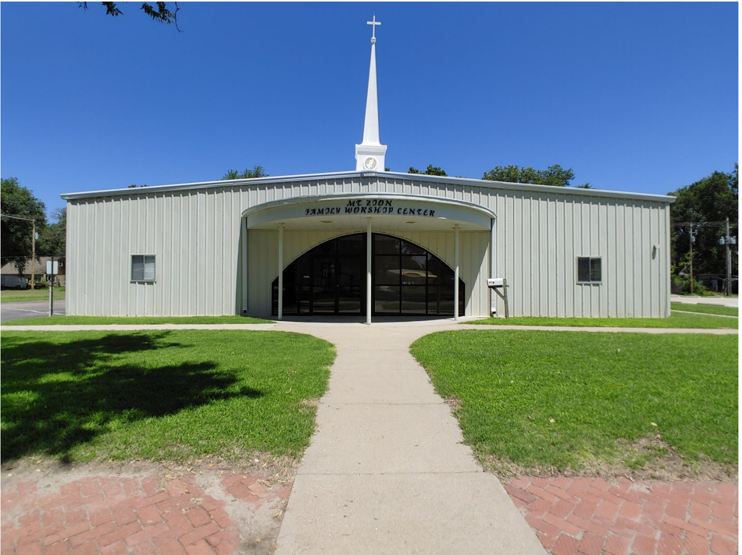
Photo 8: Mt Zion, S façade (front of building), camera facing N
