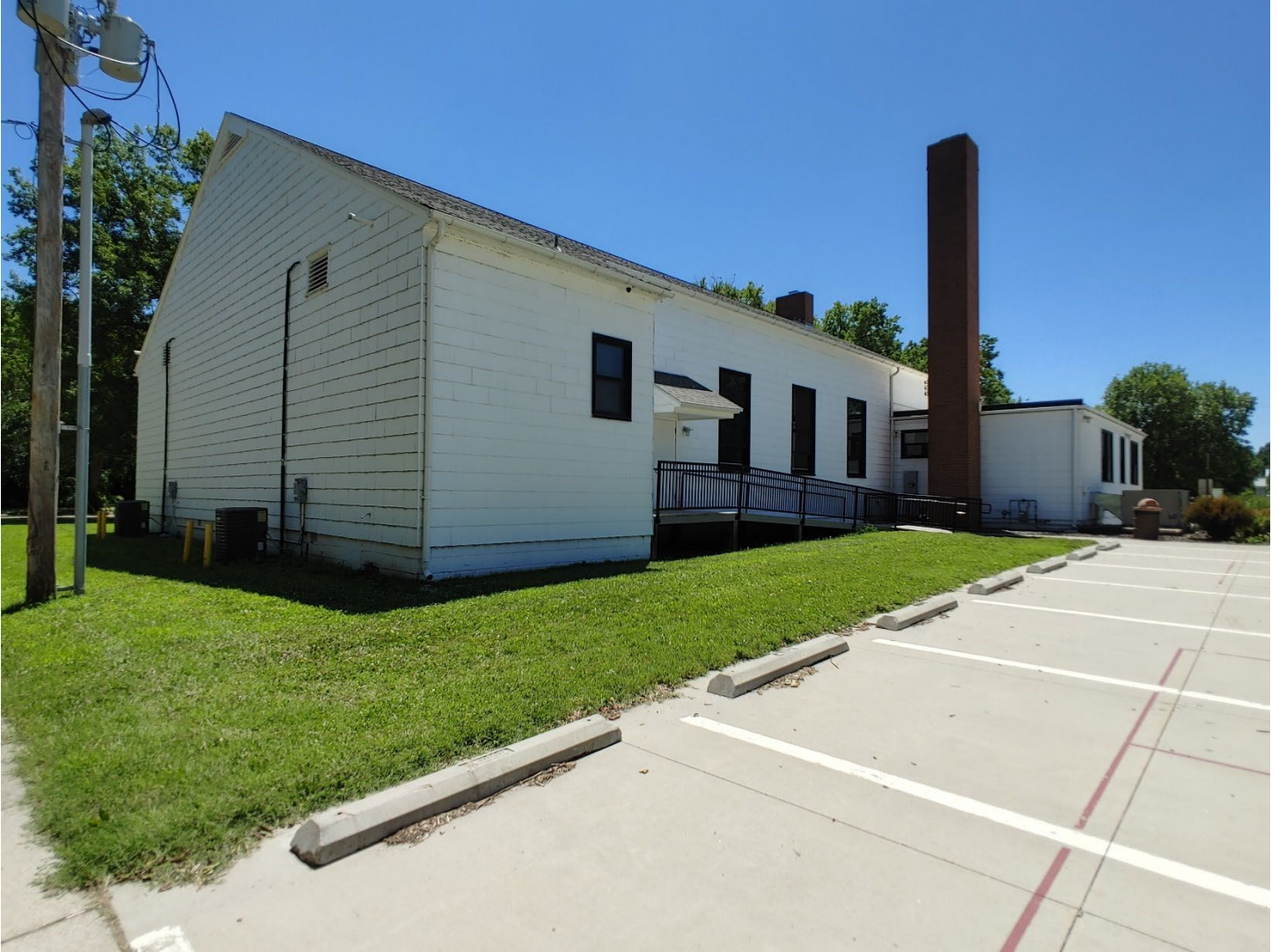
Photo 15: Douglass Community Center, NW corner, camera facing SE
