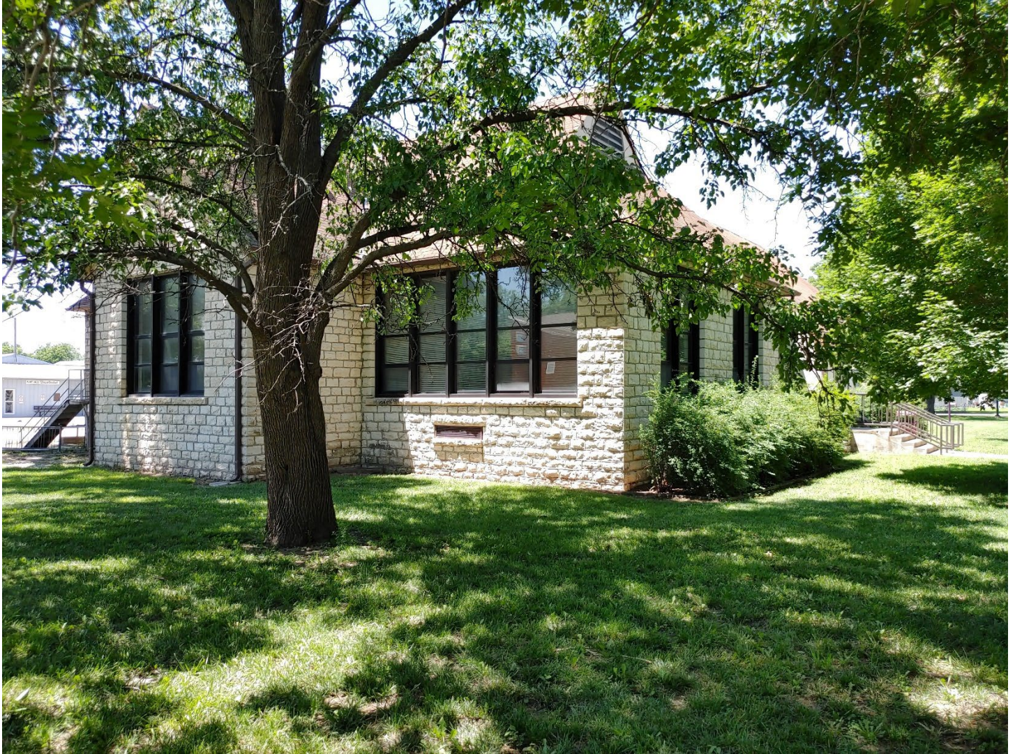
Photo 11: Douglass School, NE corner, camera facing SW
