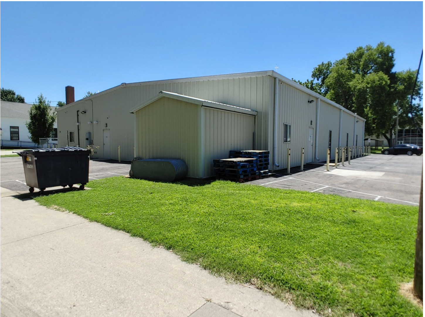
Photo 5: Mt Zion, NW corner, camera facing SE
