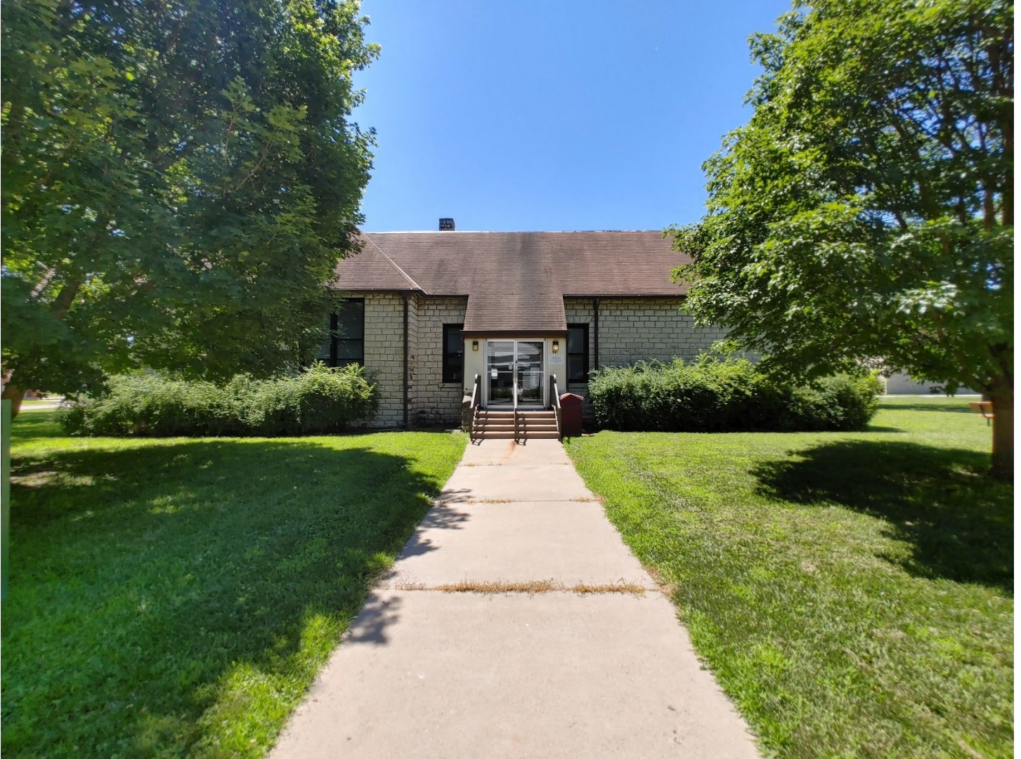
Photo 10: Douglass School, N façade (front of building), camera facing S
