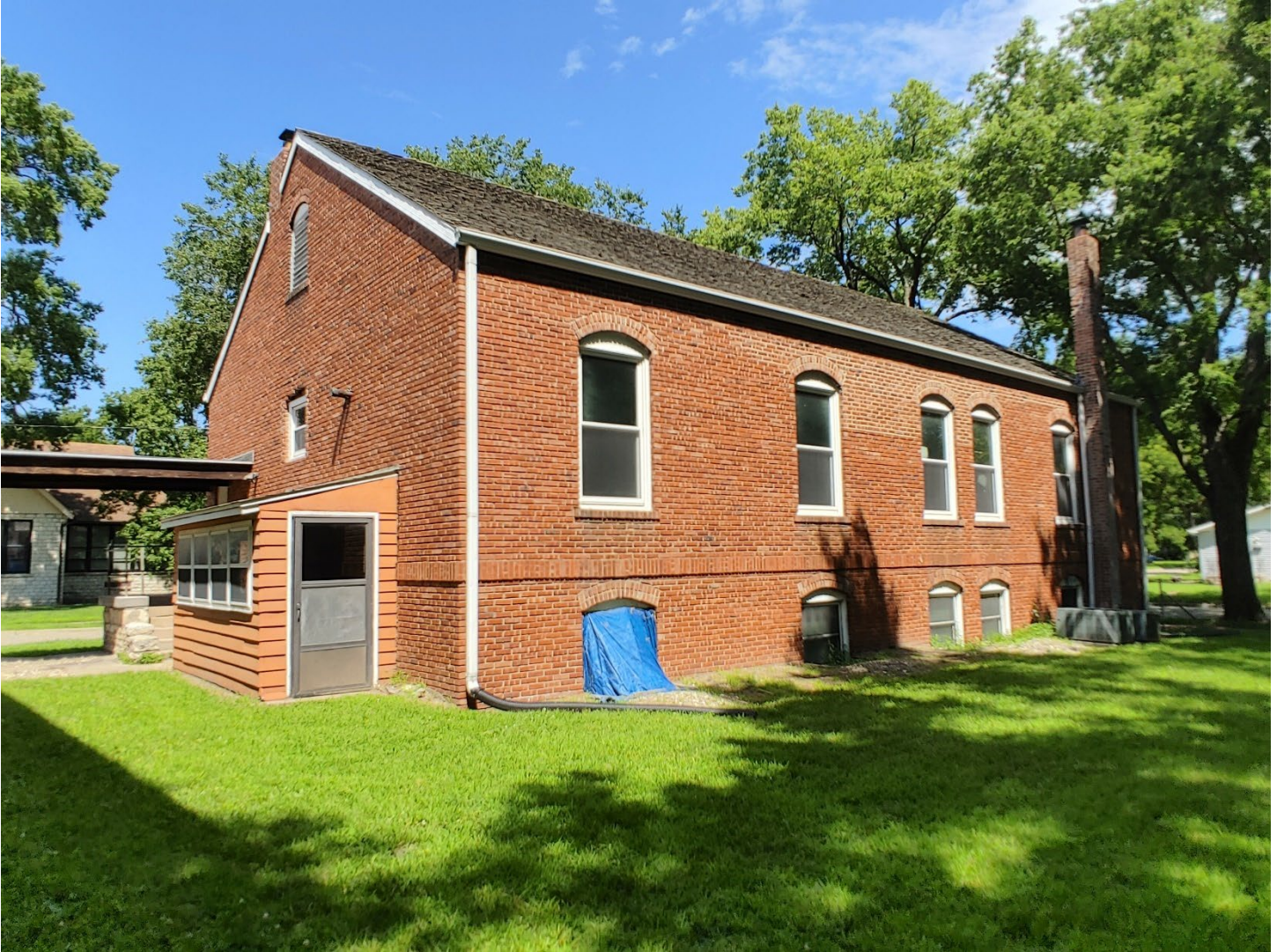
Photo 21: Pilgrim Baptist (not including addition), SE corner, camera facing NW
