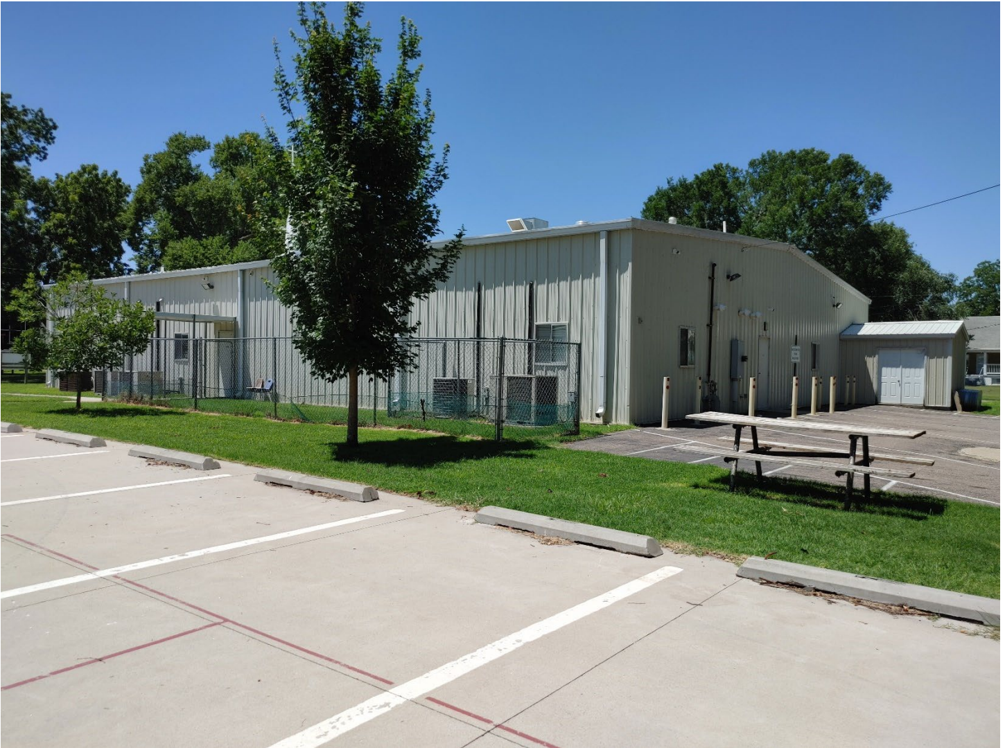
Photo 6: Mt Zion, NE corner, camera facing SW
