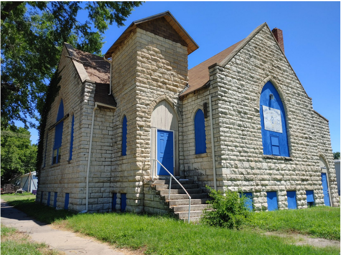
Photo 1: Shepard Chapel, SW corner, camera facing NE
