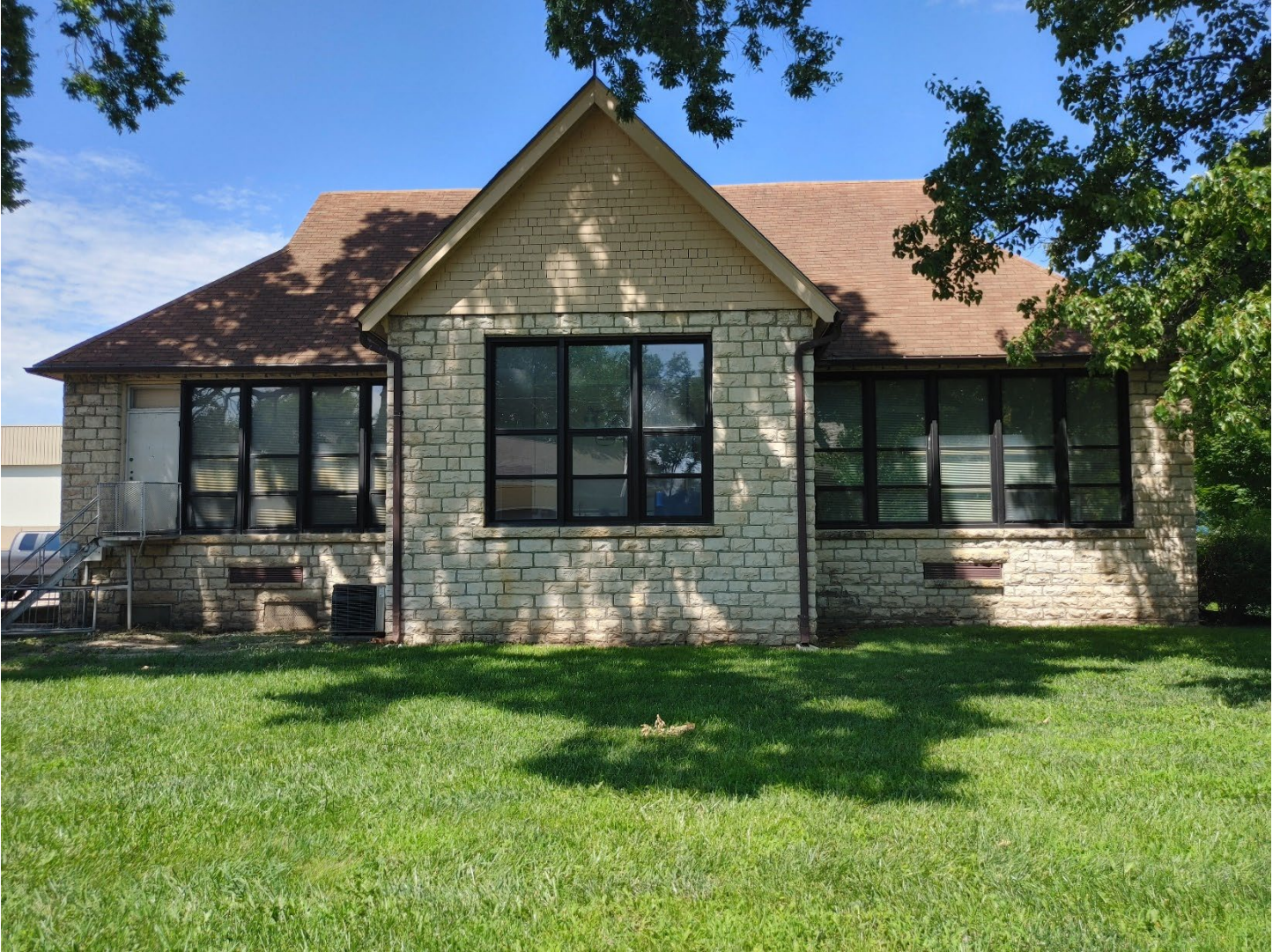
Photo 32: Douglass School, E façade, facing W
