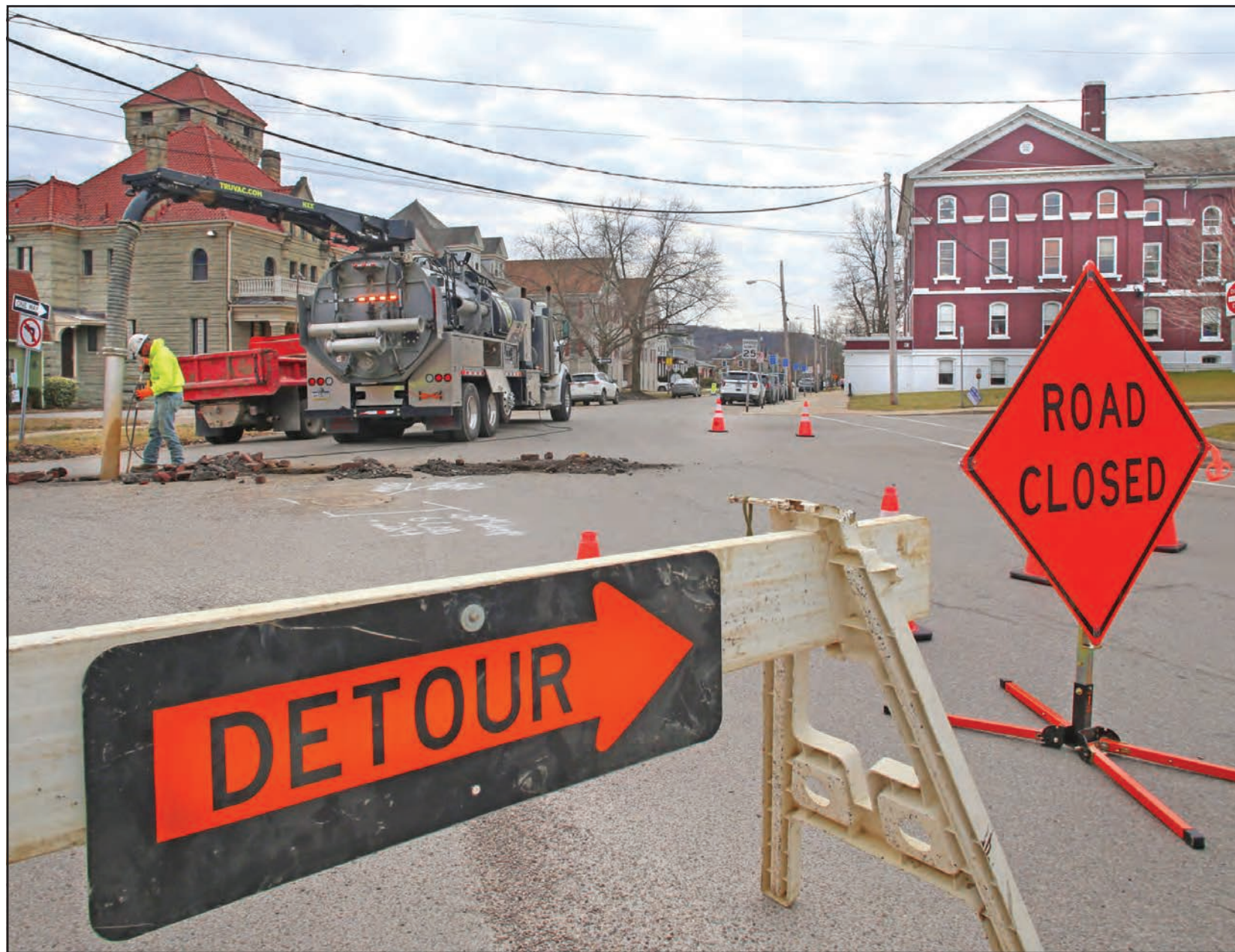
A road closure and detour sign in Franklin in March marked the start of preliminary work by Mortimer's Excavating on the city's A-108 sewer project, which stretched throughout the construction season and continues this year. Here, Matt Lockwood, of Mortimer's, uses a pressure washer and vac truck to dislodge dirt around utility lines. See the story on Page B2.
