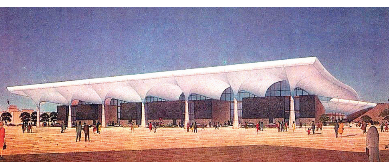
Designed by the local architectural firm of Curtis and Davis Architects and Planners, the Rivergate featured a cantilevered roof with six gently curving barrel vaults. The expressionist-style building had 130,000 square feet of meeting space.
