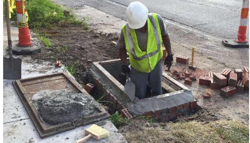
Rebuilding frame and casing of catch basin
