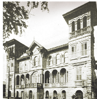
McDonogh 10 at Baronne and First streets was a school for white boys and girls. The building has been converted to apartments.
