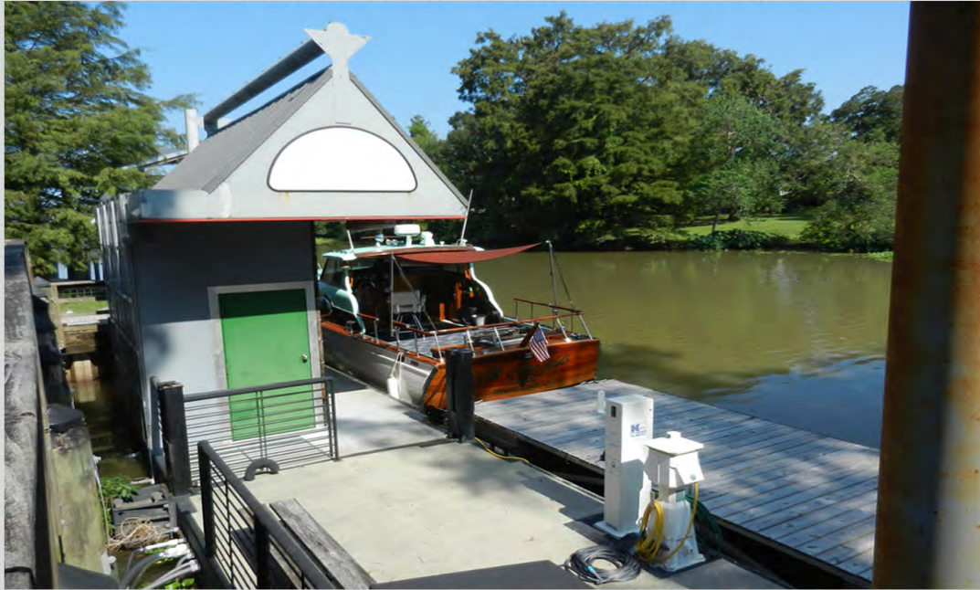
EXISTING C.V.A. TO BE RELOCATED:
