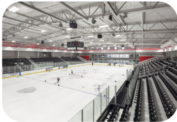
3 MidAmerican Energy Company RecPlex West Des Moines, IA
