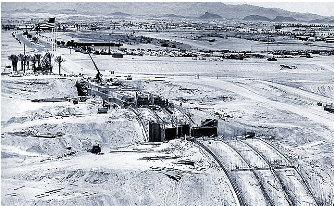
Reconstructing the bridge's arches was simplified by simply piling sand into lumps carefully piled to match the shapes needed. BBC
