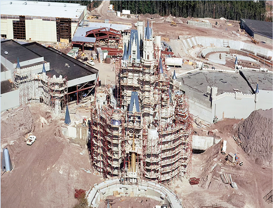
Nearly 280 tons of steel and other materials were used to build the Magic Kingdom’s 189-foot-tall Cinderella’s Castle.
