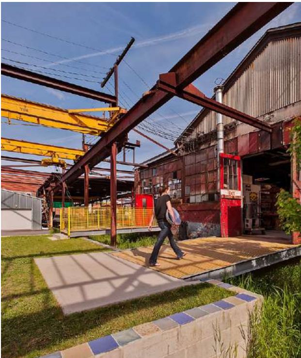
Above: Steel Yard, Providence RI
