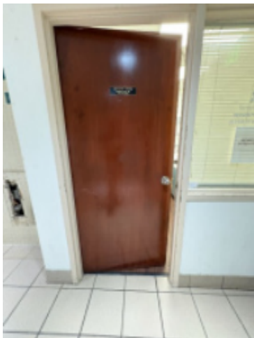
FACP signage on office door
