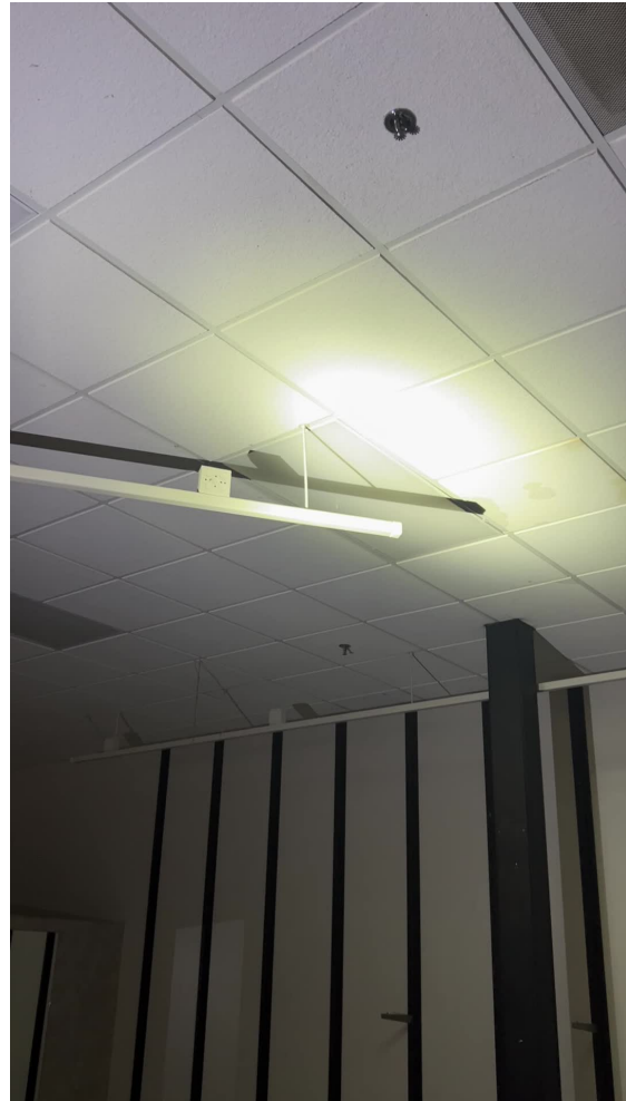
Photo 10 - Video still showing ceiling tiles and light fixtures. Source: IMG_2644.MOV.
