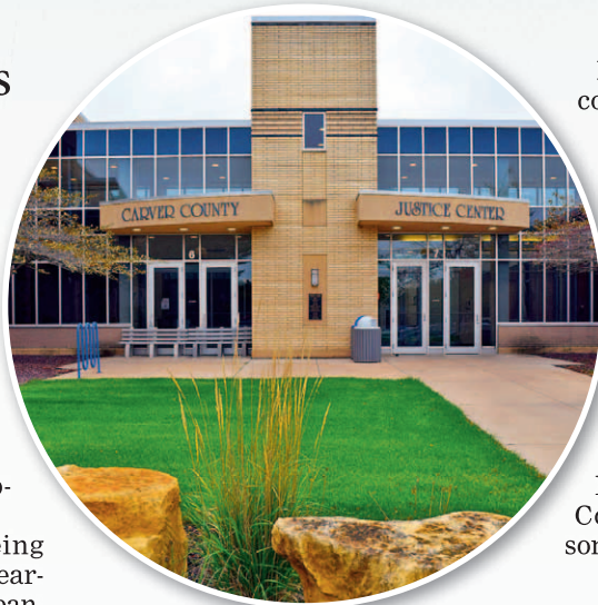
PHOTOS COURTESY OF CARVER COUNTY Carver County Justice Center
