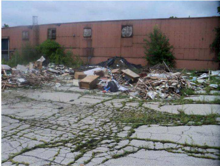
Deterioration of parking lot surface, illegal dumping creates hazardous conditions
