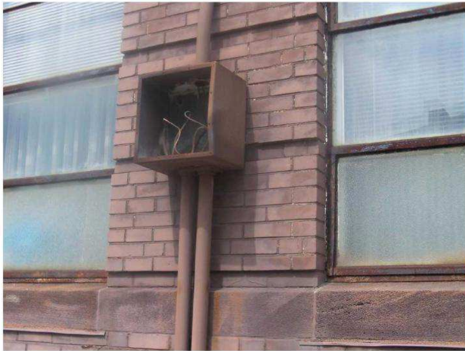
Exposed electrical wiring and deteriorated windows on Spring Avenue facade
