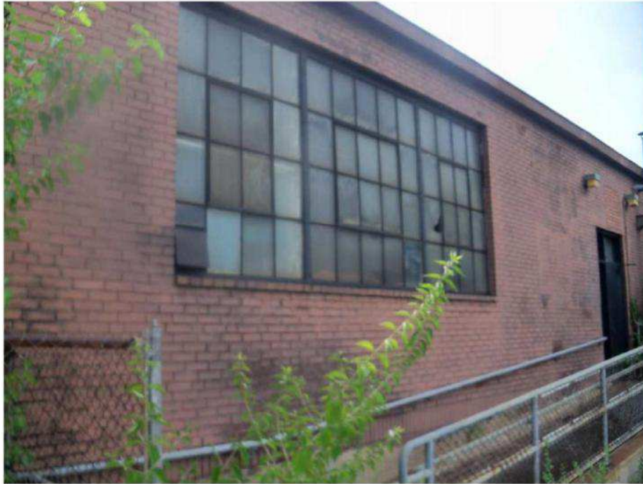
Deteriorated exterior wall and window conditions – northeast building
