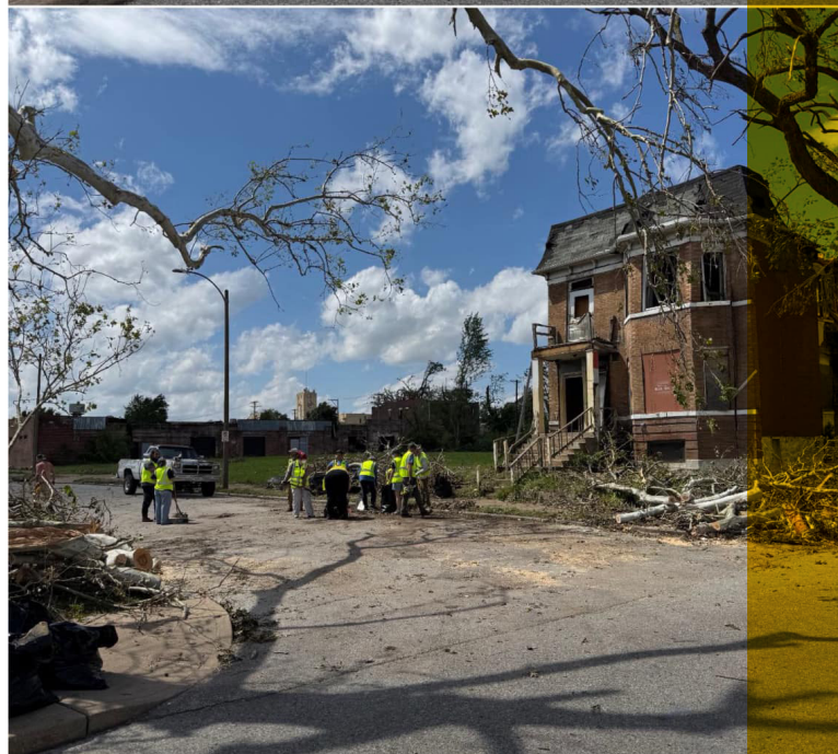
After debris removal
