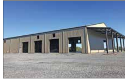
New facility for public works being built.
