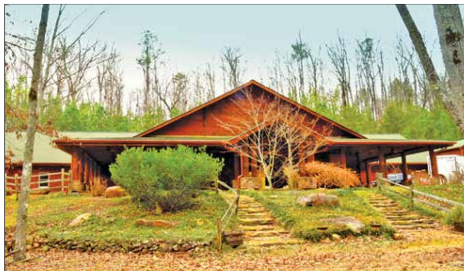
The old Lakota Cove facility is being thoroughly refurbished as a multi-purpose venue.
