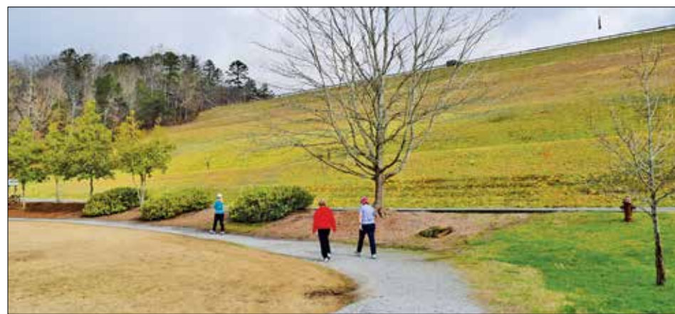
Our magnificent dam (second largest earthen dam in Georgia) provides the backdrop for exercise walkers on the playfield gravel track. PHOTOS BY ROBERT SMITH
