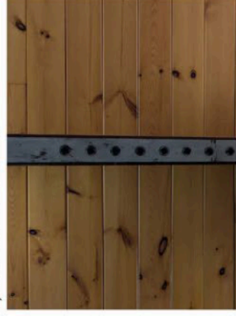
7) Metal Bracing in Classrooms
