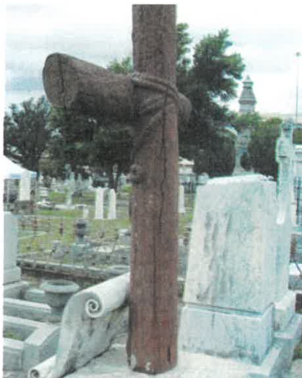
Figure 10. The sandstone cross (carved to look like wood) in this grave marker in St. Michael's Cemetery in Pensacola, FL, provides an example of inherent vice – the severe delamination affecting the sandstone has occurred along its natural bedding planes. Photo: Fran Gale.
