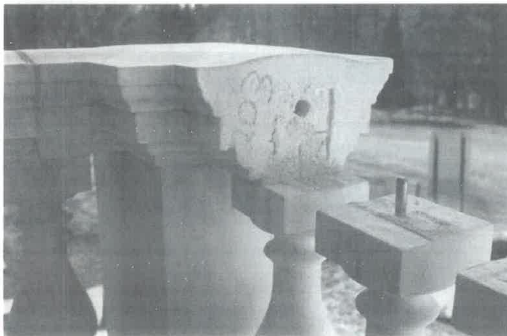
Figure 18 Long or thin cast stone elements require reinforcement. When possible, reinforcement of new cast stone should be made of stainless steel.
