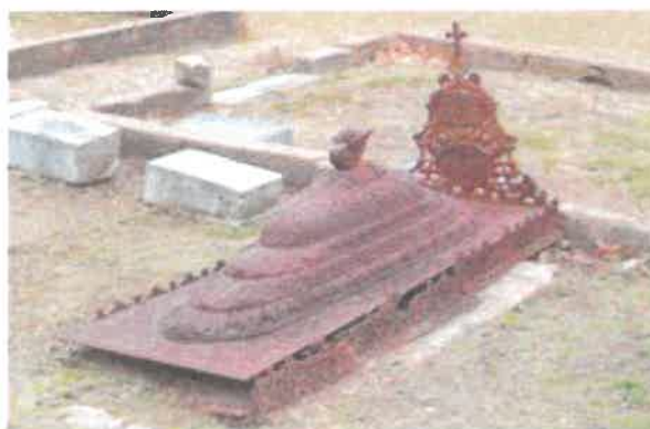
Figure 6. Decorative cast-iron grave markers like this late-19th century one in Oakland Cemetery in Shreveport, LA, are produced by heating the iron alloy and casting the liquid metal into a mold. Photo: Jason Church.
