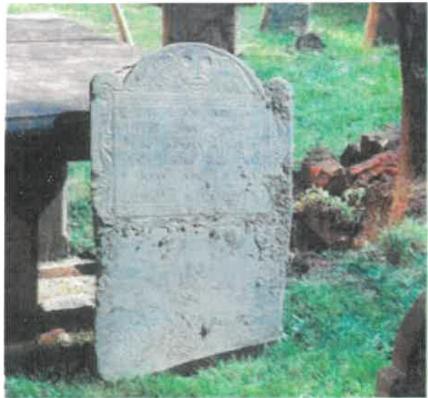
Figure 20a. This slate grave marker in the Ancient Burying Ground in Hartford, CT, is a ground-support stone. Resetting requires digging a hole that will hold the base of the stone and then compacting the soil at the bottom of the hole by hand. Photo: Fran Gale.
