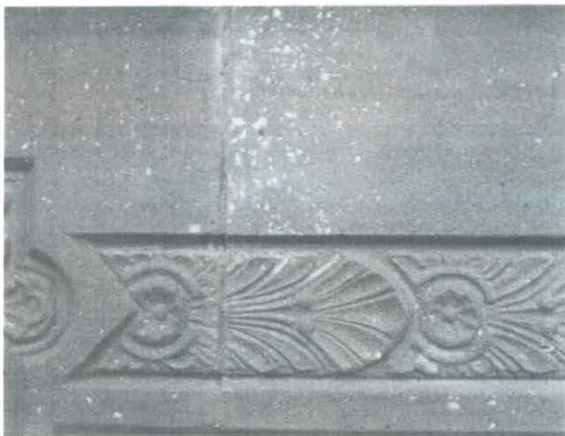
Figure 17 Unlike natural stone, cast stone generally may not be tooled in place to reduce lippage of uneven surfaces at joints. Tooling often exposes coarse aggregate from below the surface.
