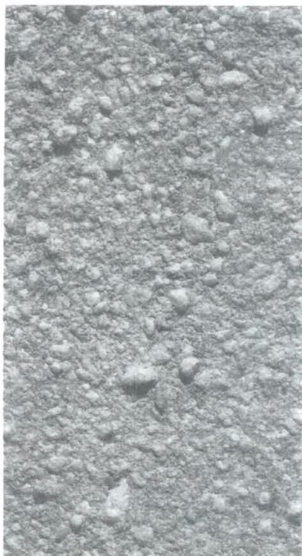
Figure 14. Sandblasting and wet grit blasting can seriously erode the surface and should not be used to clean cast stone surfaces.
