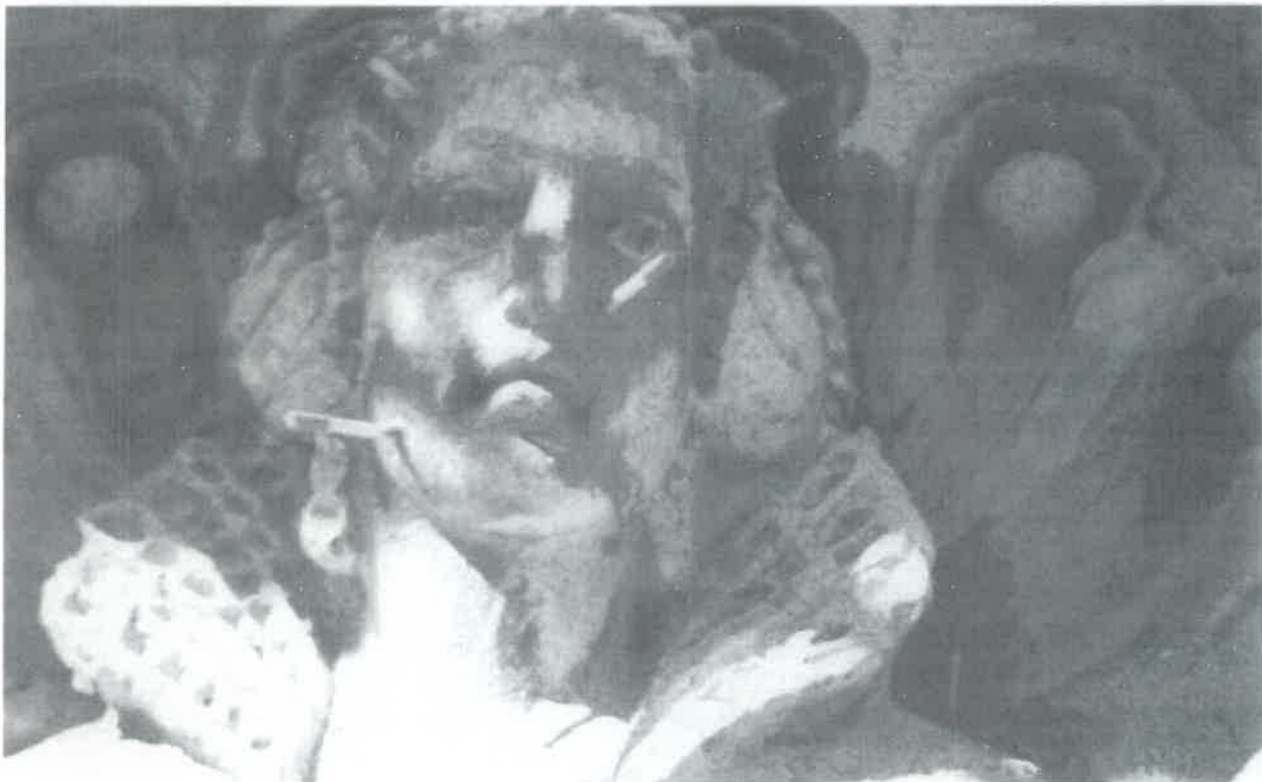
Figure 15. A delaminated layer of ornamental cast stone on the Orpheum Theater, San Francisco, California (1925), was successfully re-attached using epoxy. The multiple delivery ports for the epoxy are removed after treatment and the holes patched. Photo: David P. Wessell.
