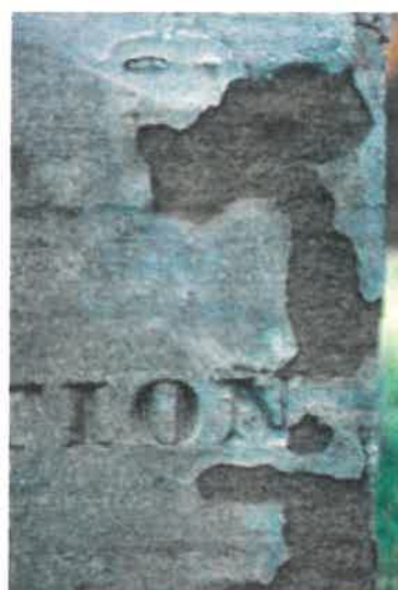
Figure 13. The impervious coating used to "protect" this sandstone grave marker trapped moisture within the stone, eventually resulting in deterioration and surface loss. Photo: Fran Gale.
