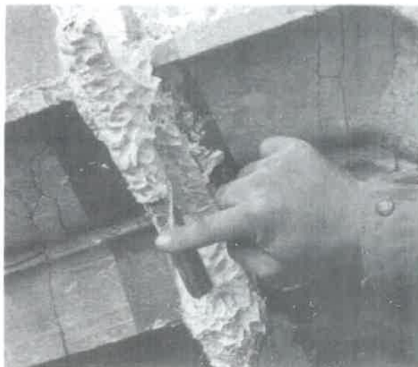
Figure 19. Molds for the replication of cast stone may be made on site using rubber materials and reinforcement. The molded profile of this window pediment will be used to run a plaster mockup, from which a production mold will be made. Photo: Michael Deconshire
