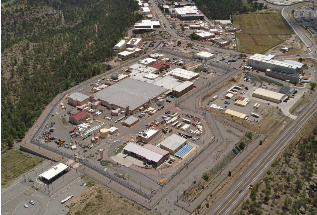
Figure 2.4-1 PF-4 in TA-55 (Looking Southeast)
