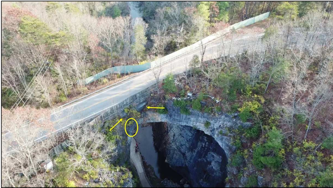
Figure 6. Still image from RU UAS video looking downstream from the north. Shows orientation of Route 11 crossing Natural Bridge at oblique angle and proximity to sensitive features. "Old Man" structure is circled. Arrows indicate concrete buttresses placed in 2000 to reduce erosion and undermining beneath the pavement.
