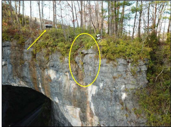
Figure 8. Still image from RU UAS video. Close-up of sensitive area of rock on the downstream-side of the rock formation. Low safety factor block is circled. Arrow indicates loudspeaker used during nightly sound-and-light shows.
