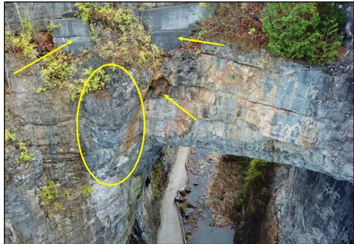
Figure 7. Still image from RU UAS video. Close-up of sensitive areas of rock structure below the roadway. "Old Man" structure is circled. Arrows indicate solution void opening and concrete buttresses placed in 2000 to reduce erosion and undermining beneath the pavement.
