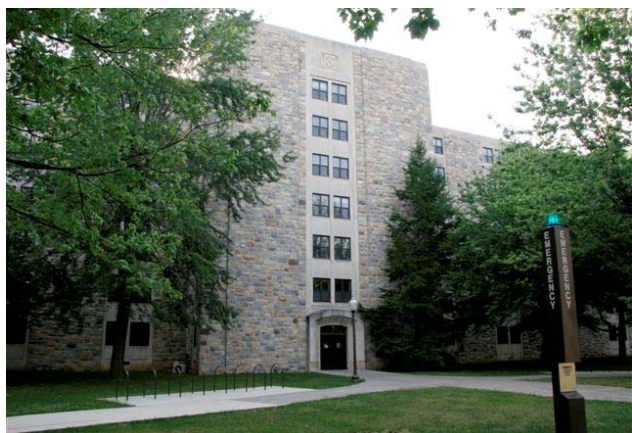
Figure 3. Exterior of West Ambler Johnston
